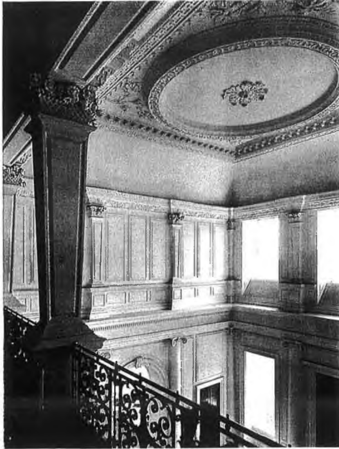
Fig. 16 The upper part of the entrance hall.
