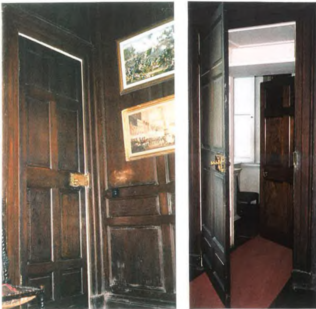
Fig. 27 The doorways in the brown study, note the original panelling and the difference between the 1720s and 1760s doors (right).
