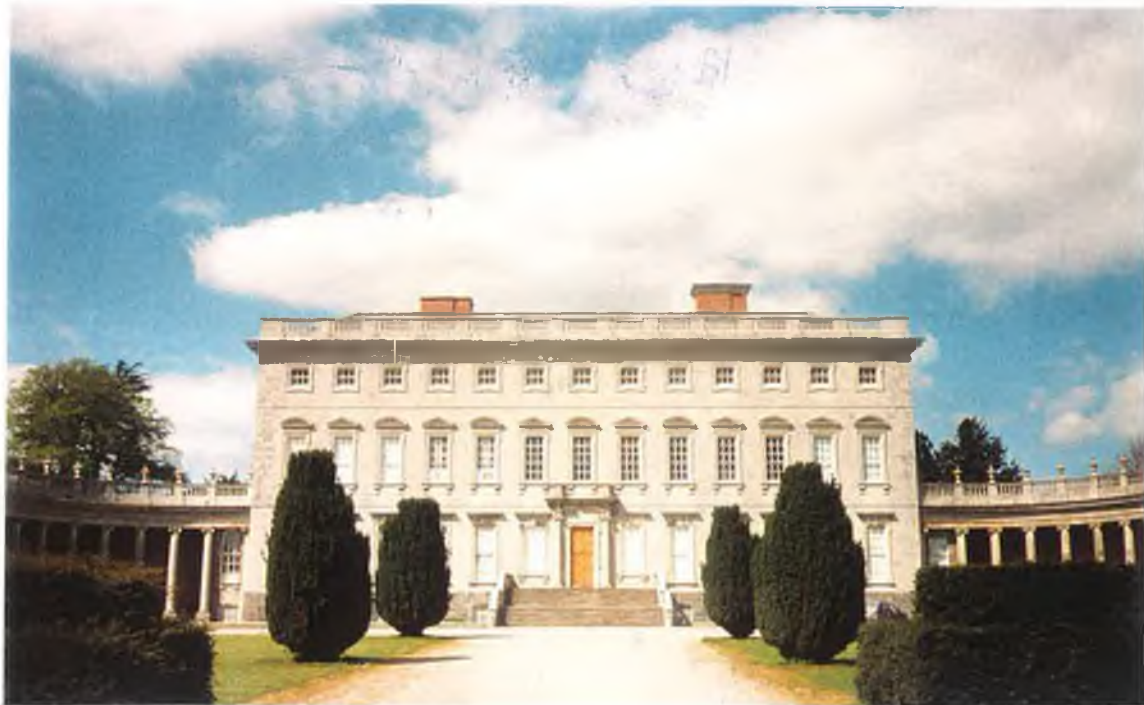
Fig. 7 View of the central block of Castletown.
