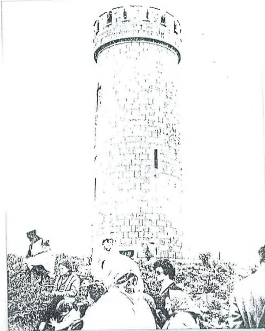
Fig. 12. Tower on Hill of Allen.
