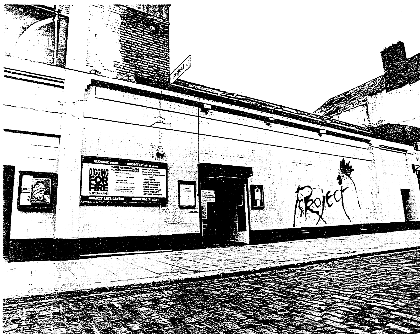
PHOTO 2 The Project Theatre Company's building, before redevelopment.
