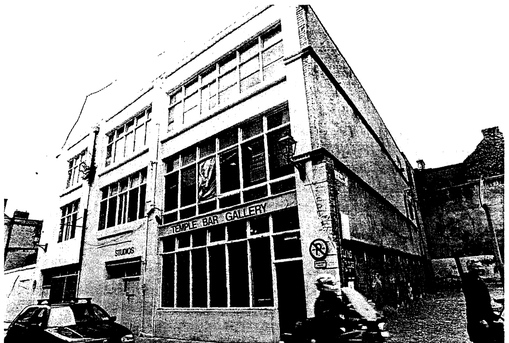
PHOTO 1 The Temple Bar Gallery and Studios, before redevelopment.
