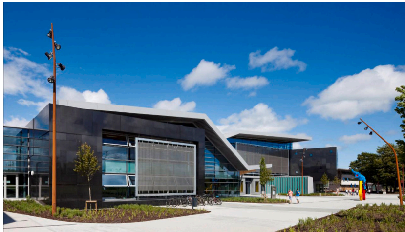
Fig. 3. SLLS building located at University College Dublin, Ireland.
