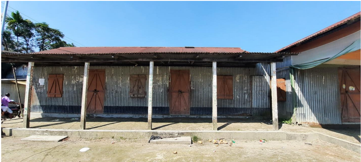
Image n. Baghbar Bazar Committee house
