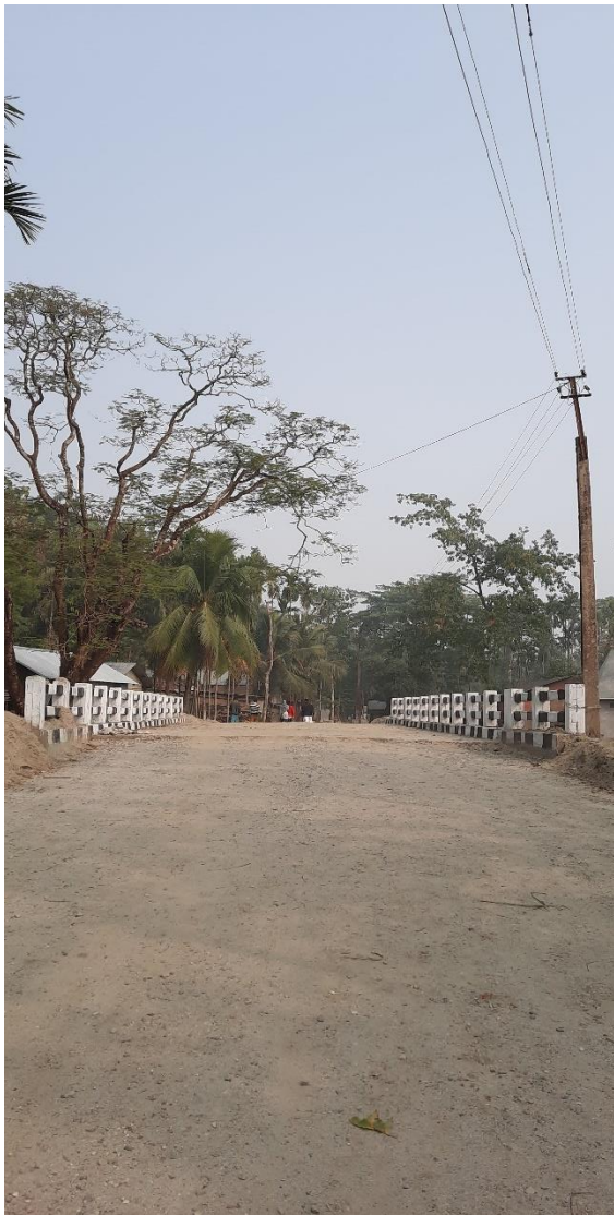
Image j. A newly constructed RCC (Concrete) bridge at Baghbar Pahar.
