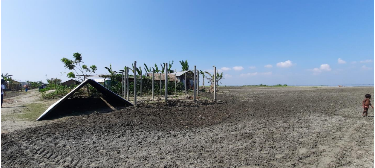
Image r. A house being shifted, the tin walls have already been taken, what is left are the tin roofs and the concrete posts.
