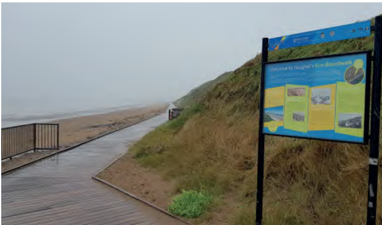
Figure 9.6 The Youghal boardwalk in County Cork destroyed in storms in 2014 (top) and rebuilt in 2019 (bottom). Credit: John Finn and Smith et al., 2022
