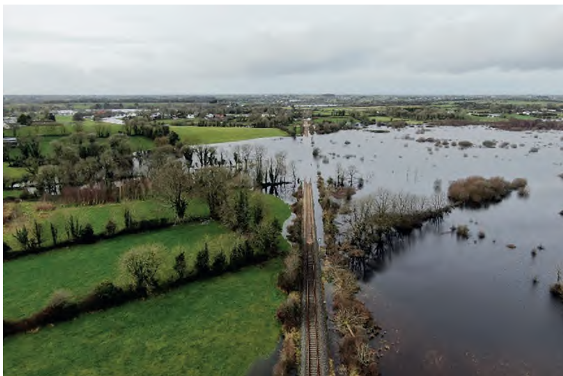
Box 5.1 Figure 1 Groundwater along the western railway corridor near Gort, Co. Galway, in winter 2020. Photo credit: Galway County Council.
