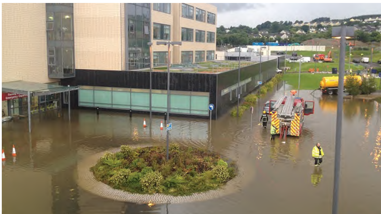
Figure 8.4 Letterkenny hospital after floods in 2013, when 40% of hospital services had to be taken out of clinical use. (Source: McGinley (2014), Photo Declan Doherty)
