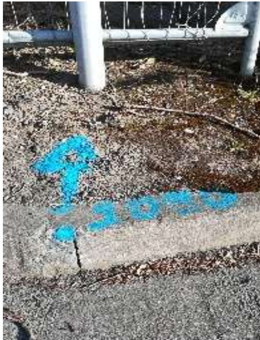
Plate 5.8: Marking of the culverted river Poddle as a 1050mm surface water drain on the construction site of the new build-to-rent development (Plate 5.7) (Source: Author, 2022)
