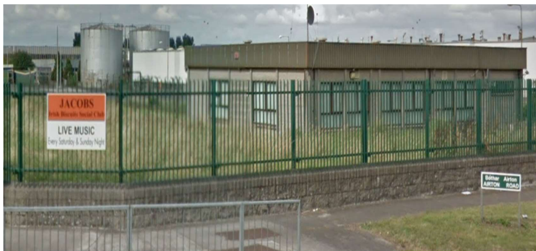
Plate 5.3: Photograph of the social club before its demolition (Source: Google Maps street view, 2014)
