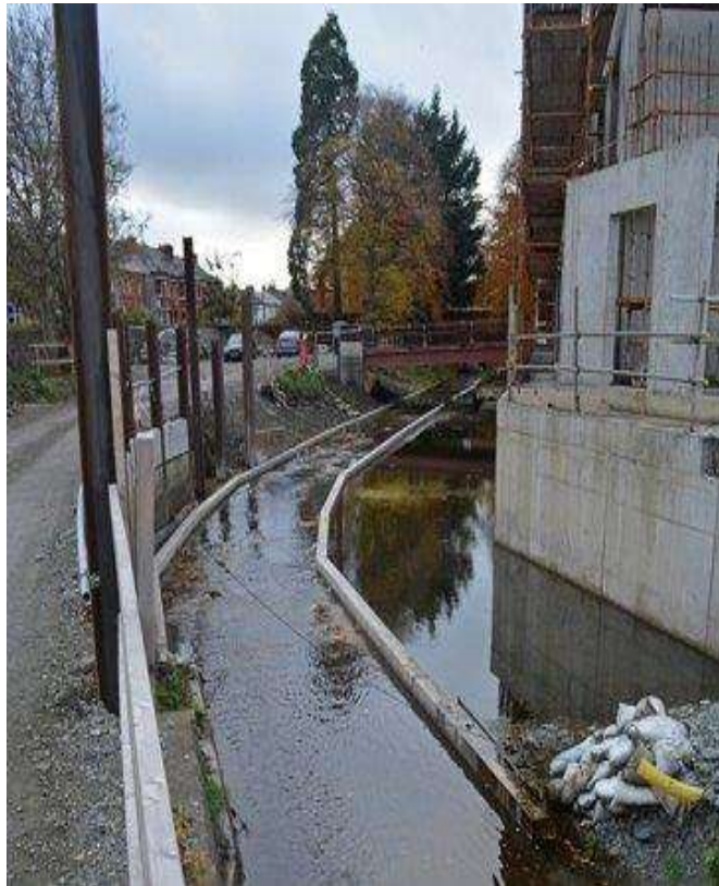
Plate 4.4: Luxury build-to-rent development and its river Poddle channel realignment (Source: Krystallas, 2017)
