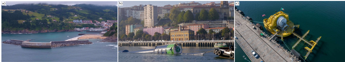
Figure 2.3: Examples of the three main types of OWCs: a) Mutriku wave power plant, Basque Country, b) IDOM Marmok-A5 spar-buoy, and c) OceanEnergy OE35 BBDB. Source: [51].
