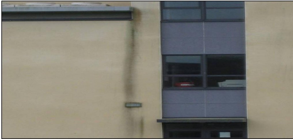
Figure 5.4 Building façade discoloured by excess surface water not managed by drainage provisions.
