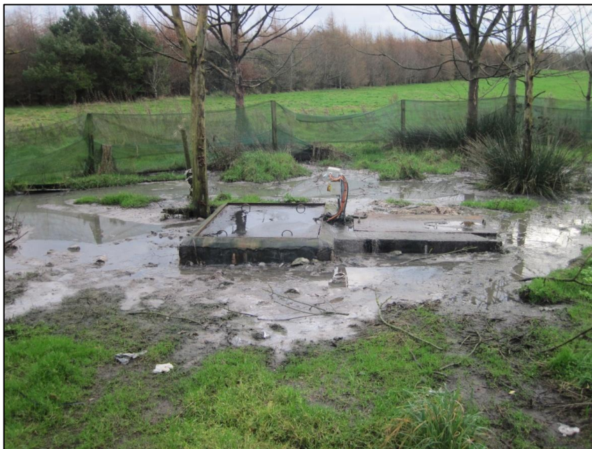
Figure 4.2 Legacy septic tank sump overflow in a low permeability setting. (Source: Limerick County Council, 2011.)
