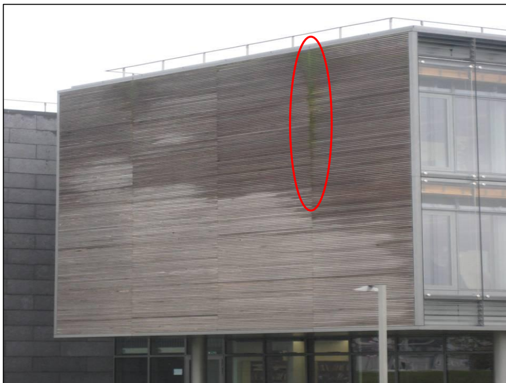
Figure 3.3 Wind-driven rain on two-year old cladding. Green mould is growing in the vertical seam towards the top-right, circled.
