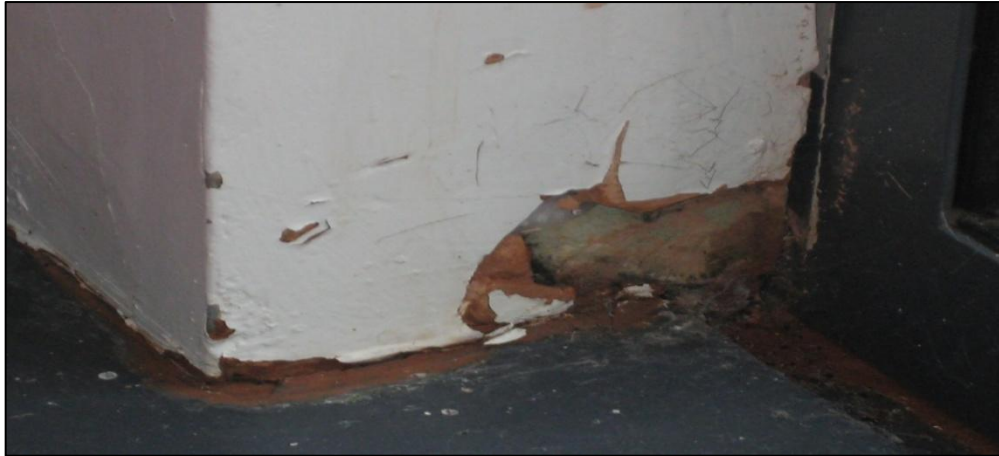
Figure 3.2 Interior damage due to wind-driven rain penetration. Damp can be observed at lower right.
