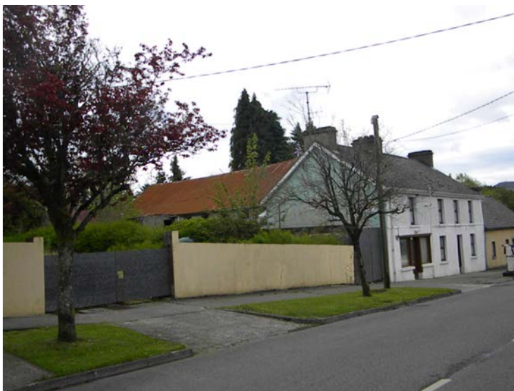
Fig. 5.6 McGowan Dance Hall and Cinema (white structure and two-story building with red roof behind) now empty in Kiltyclogher, Co. Leitrim. source: photograph by author.
