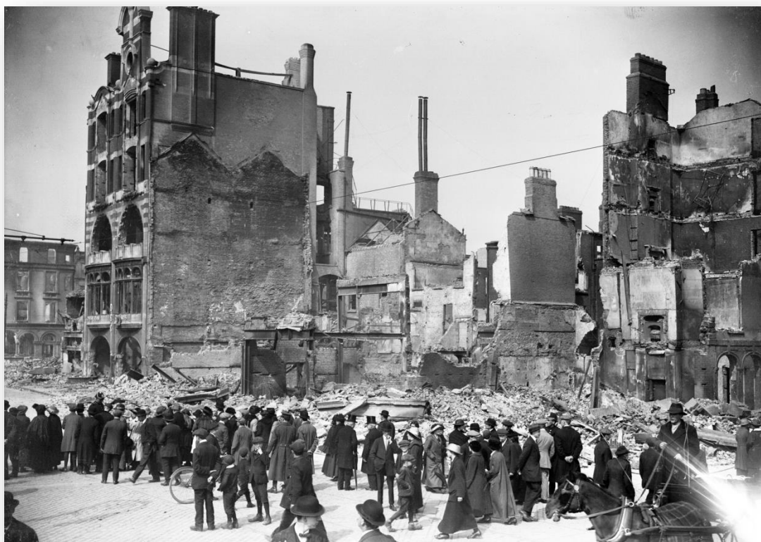
Dubliners view the ruins at the southeast corner of Lower O'Connell Street after the Rising. The large building on the left of the image is the DBC (Dublin Bread Company tearooms) and to the left of it are the remains of the Grand Cinema. Image courtesy of the National Library of Ireland
