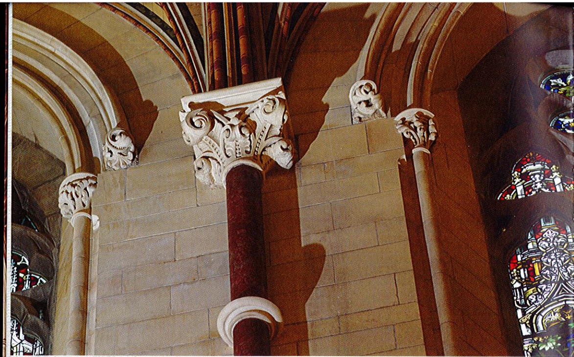
Buttressed window divisions with Caen stone on interior walls
