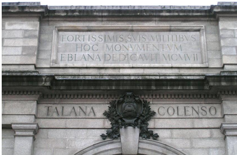
Fig. 66: A modern photograph of the front of Fusiliers' Arch.
