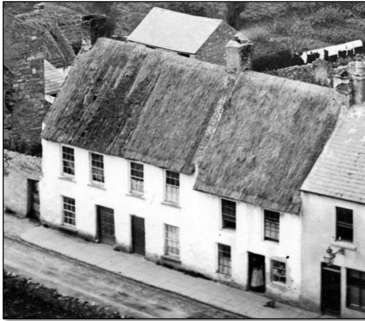
Figure 4.8 An example of the type of two-storey thatched town house, which was probably typical of much of the better-class urban housing fabric of Sligo through the 18 th and early 19 th centuries. These buildings, along the northern side of John Street, survived until about 1899. The dwelling to the right has already converted its thatch to slates. Source: NLI, Lawrence collection, STP. 1047, (extract).
