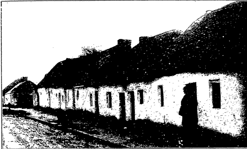
This is a view of houses of the poorer classes at Duck Street, Sligo. Weekly tenants.
