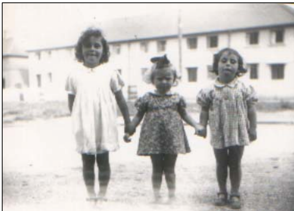
Fig. 7.17. The Jenkin's sisters, Charlotte Street, Sligo, ca. 1938. Waiting to move into the new Abbeyquarter scheme, under construction in the background. Courtesy, D. Foley, Sligo.
