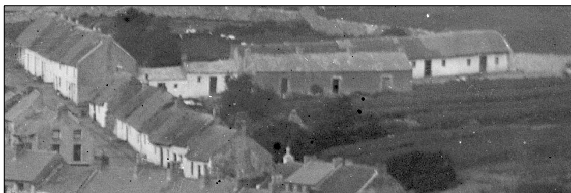
Fig. 5.6 The King Street houses, ca. 1899, also showing the houses on the east side of Holborn Hill. Source: Lawrence collection, NLI, extract from LCAB 05637-15602.
