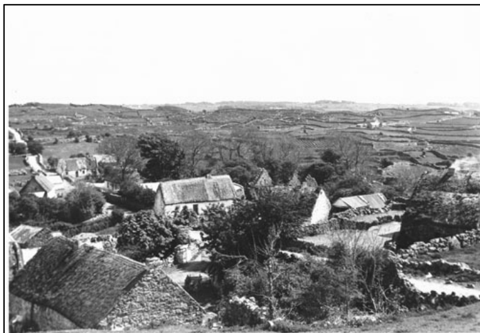
Figure 7.21. Photo of old cottages at Shantalla, Galway in 1946. Photos, National Museum of Ireland, by P. Mac Dúbháin.
