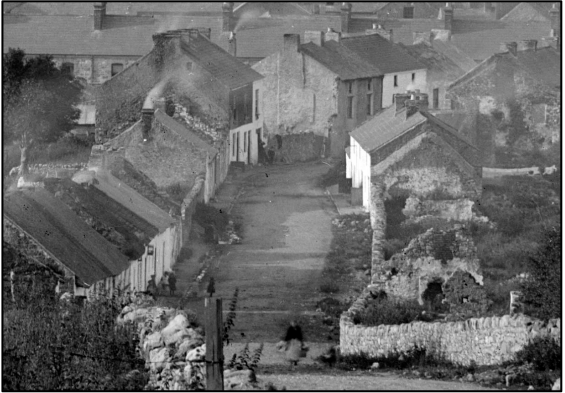
Fig. 5.13. Photo of houses South Gallows Hill, Sligo, c. 1900. Source: NLI, Lawrence Collection , LCAB 3271. (Enlarged extract).
