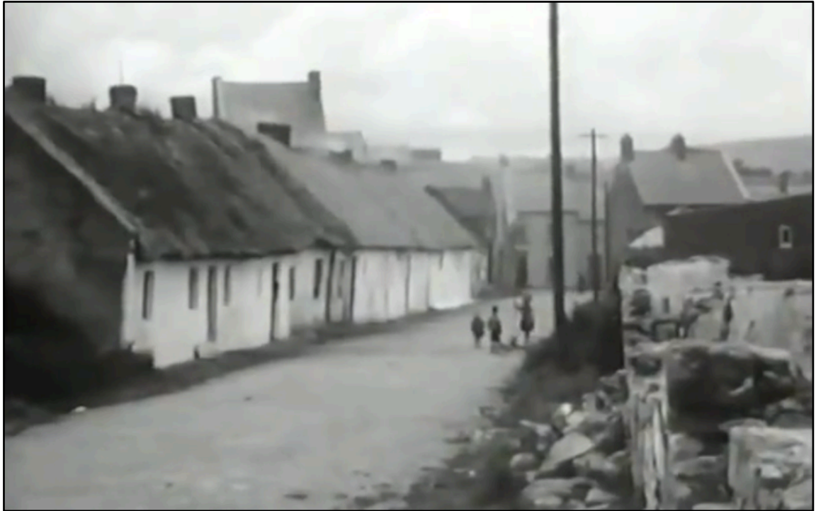
Figure 6.15. Some of the houses on The Ropewalk, (Vernon Street), in 1935, shortly before demolition. Source. Author's collection.
