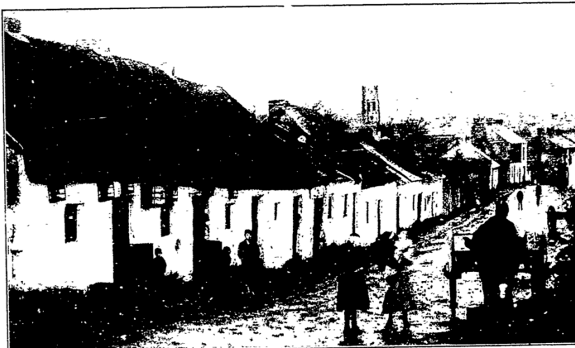
This is a view of houses of the poorer classes at South Gallows Hill, Sligo. Weekly tenants. Reading from left to right on the photograph—
