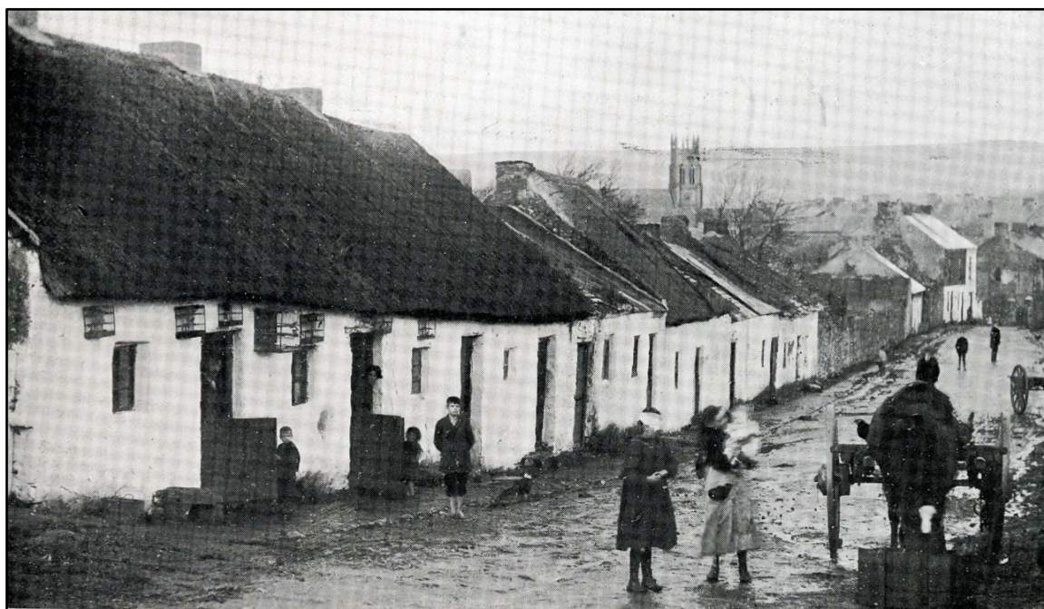
Fig. 5.11. Photo of poorer-class houses at South Gallows Hill, Sligo, 1913, west side. Source: Appendix to the report ..... HC 1914 [Cd. 7317], appendix xxxvii, p. 391/501.
