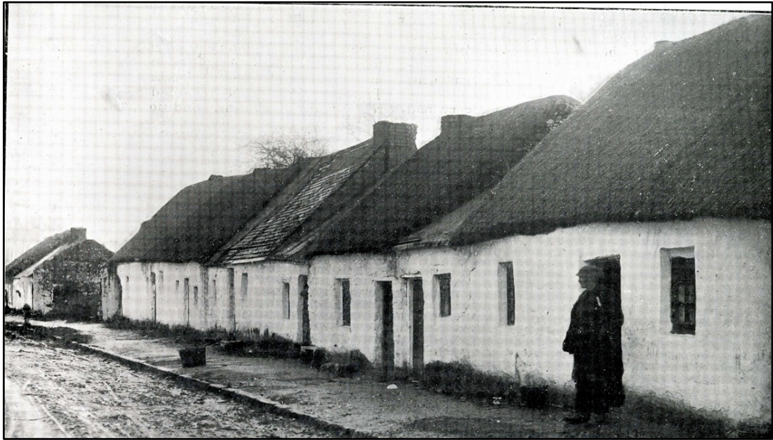
Fig. 5.8. Photo of houses at Duck Street, Sligo, 1913, south side. Source: Appendix to the report ..... HC 1914 [Cd. 7317], appendix xxxvii, p. 388/500.
