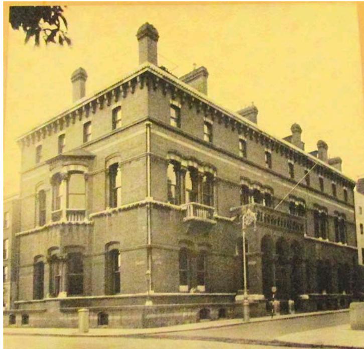
Figure 6.3 Kildare Street Club (after 1860). Kildare Street and University Club Archive.
