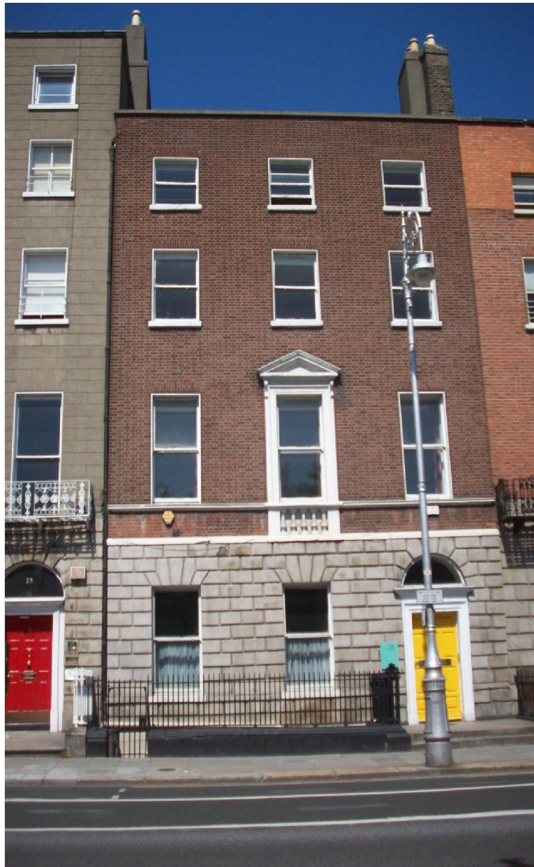
Figure 30.1 No. 26 Merrion Square North
