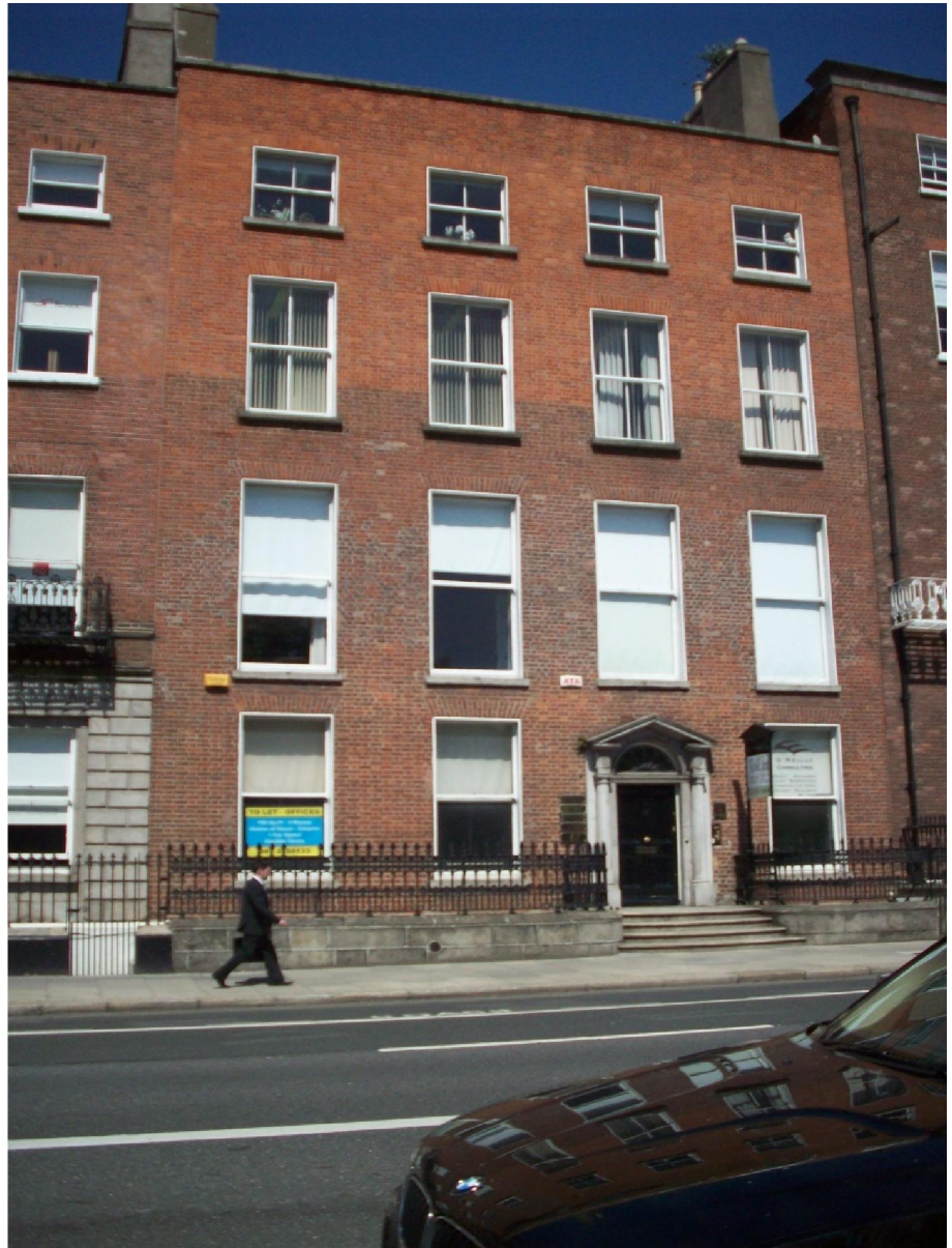
Figure 29.1 No.11 Merrion Square North
