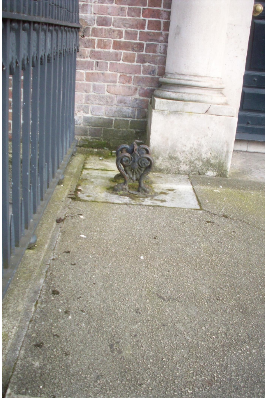
Figure 31.13 No.45 Iron work
