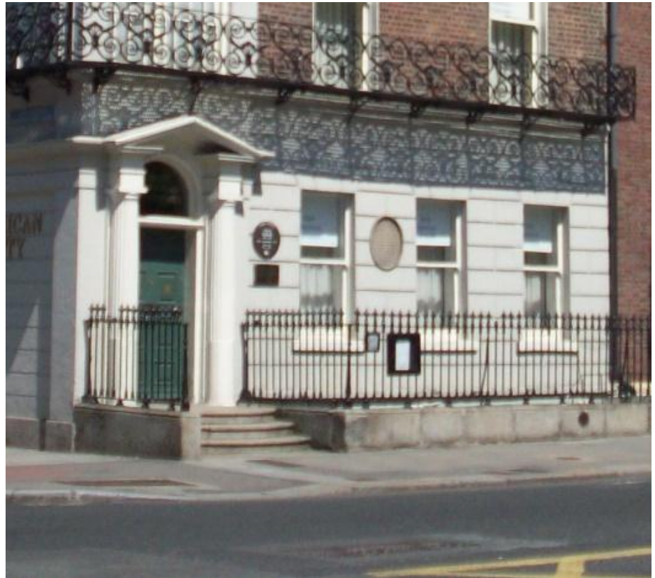
Figure 28.2 No.1 Merrion Square North front brick work
