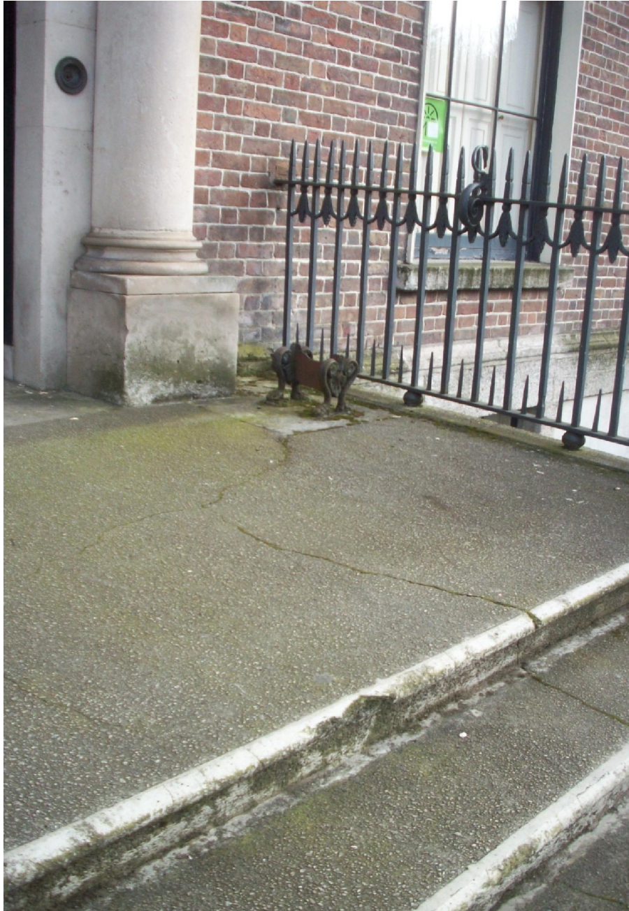
Figure 31.2 No.45 Iron work
