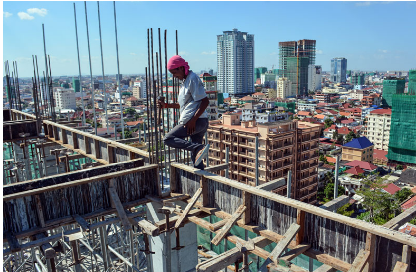
Figure 1-2: Construction Worker on Site in Cambodia (Consiglio, 2014)
