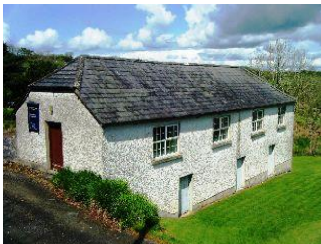
Figure 2.2 Ervey Presbyterian meeting-hall, completed 1807
