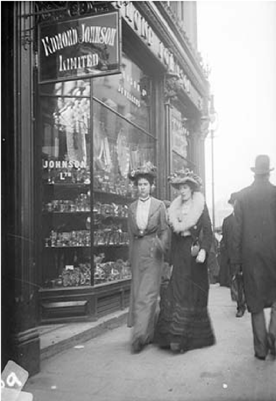
Figure 6.7 Edmond Johnson Limited shop exterior, photographed c.1897-1904?
