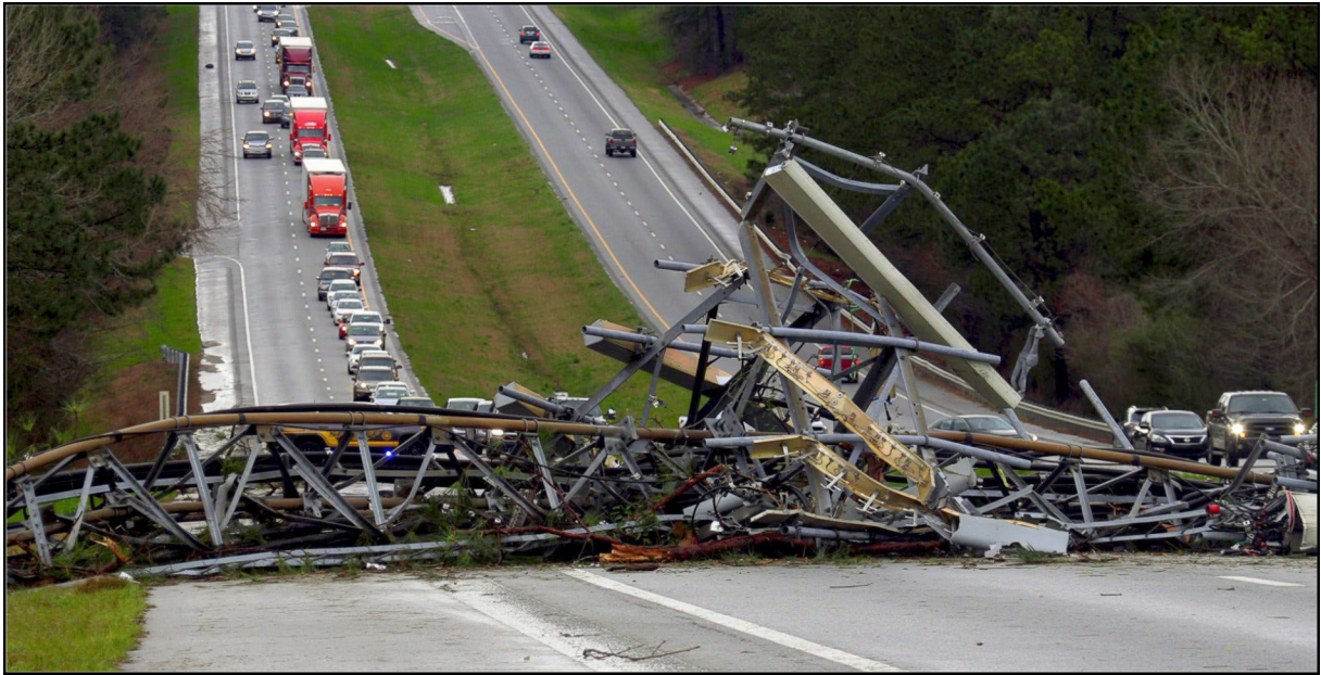
FIGURE 1. Disaster-struck cell tower [14].
