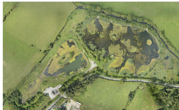
(b) Maynooth Reservoir.
