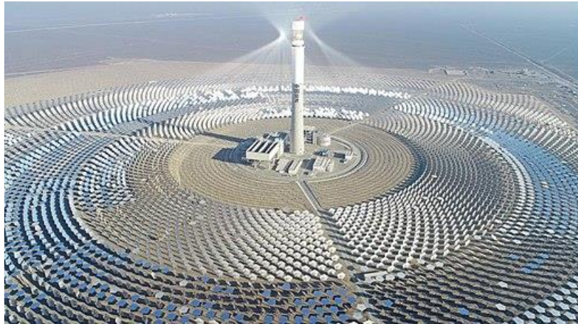
Figure 14. 50 MW high temperature molten-salt power tower in Hami, China (credit: Csp.guru, CC BY-SA 4.0 < https://creativecommons.org/licenses/by-sa/4.0/ >, via Wikimedia Commons)
