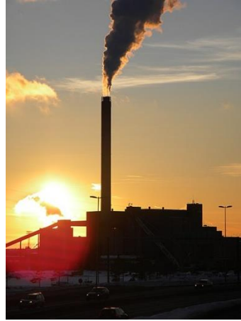
Figure 49- Salmisaari CHP power plants by sunset in Helsinki, Finland — (credit: Pöllö, CC BY 3.0 , via Wikimedia Commons)
