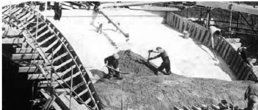
Spreading the concrete at river Ouse viaduct. Source: John Laing archive
