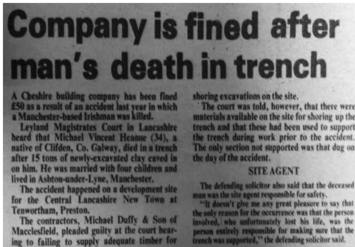
Figure 4.10 – Trench Collapse – (Source: Irish Post , 29 January, 1977, p.7.)
