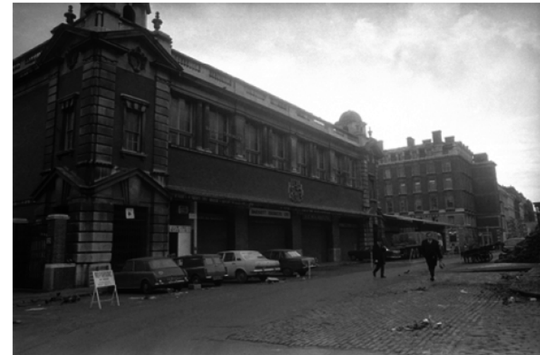
Figure 1 - Covent Garden c.1973 (photo Copyright © 2010-2018 New Video Channel America, LLC)
