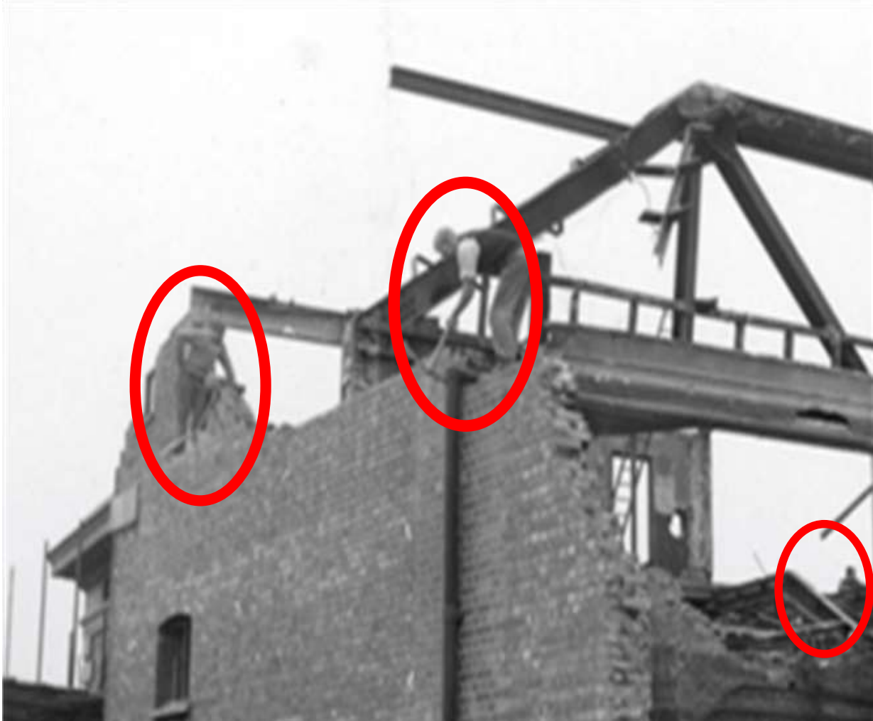
Figure 4.11 - Demolition of Chiswick Empire - west London, 1959.
