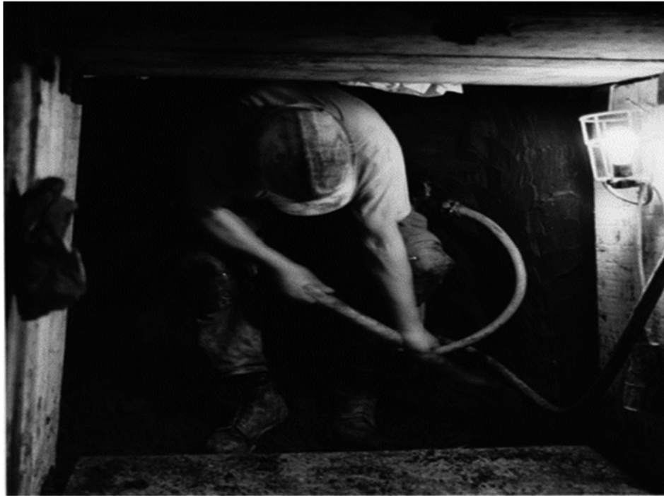
Figure 3.6 - a typical public water sewer connection tunnel being excavated by hand (Source: Timothy O’Grady & Steve Pyke, I Could Read the Sky , (London, 1997), p69.)
