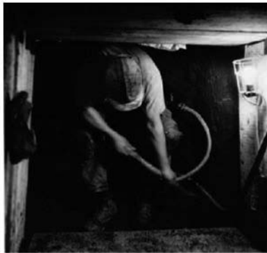
Figure 1 - a typical sewer connection tunnel being excavated by hand (Source: Timothy O'Grady & Steve Pyke, I Could Read the Sky , (London, 1997), p69.)
