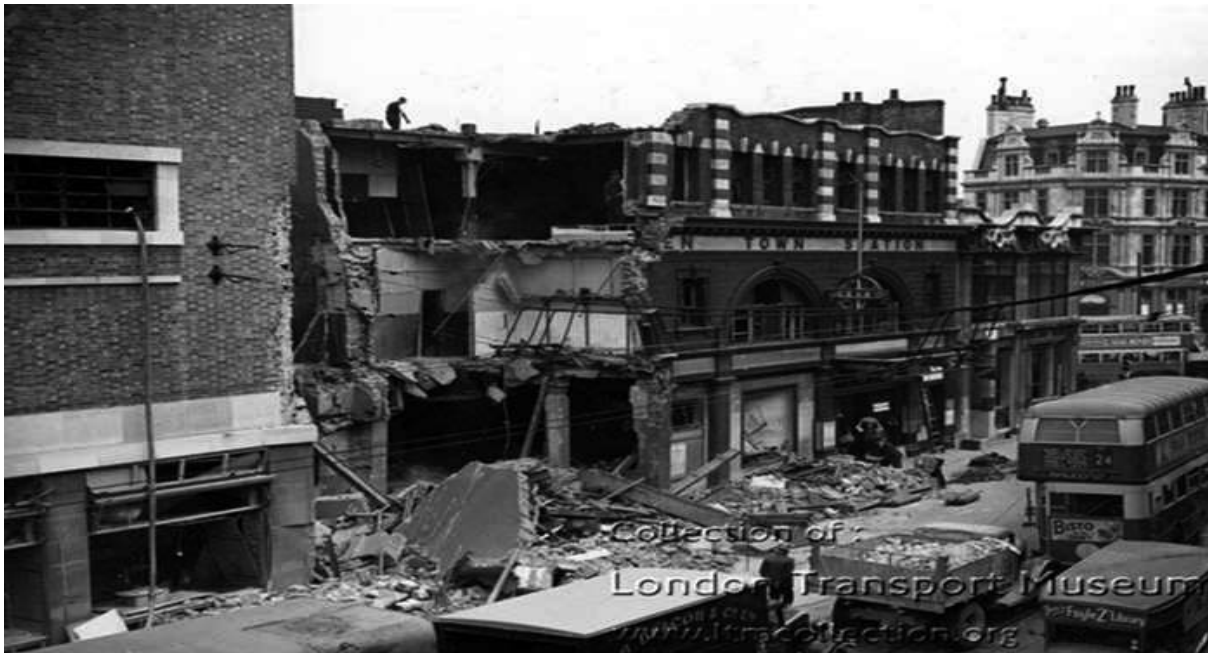
Figure 5.9 - Camden Town Underground station, Northern line. Exterior view showing bomb damage sustained to the Camden High Street facade of the station.
