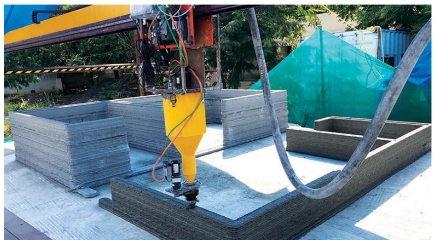
Volumetric (3D) Concrete Printing Technology (VCPT)
