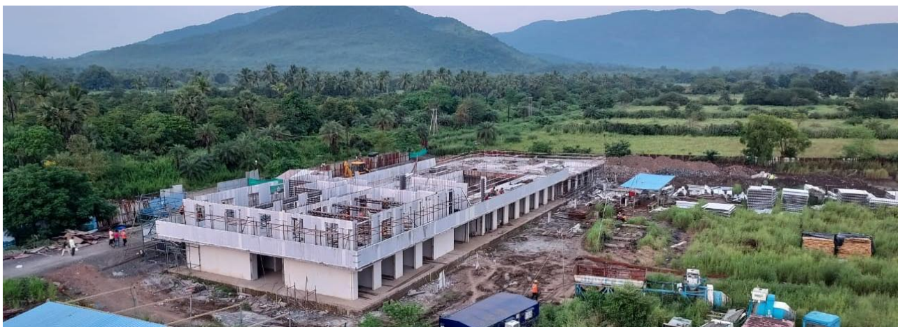
Building under Construction using PVC “Stay in Place Formwork”
