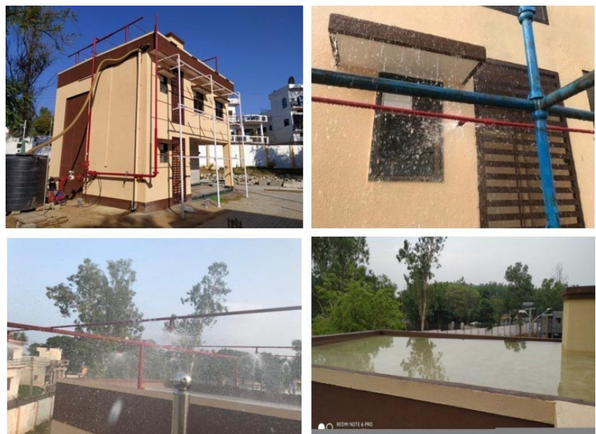
Fig. 5. Actual water testing setup facility in AAC building
