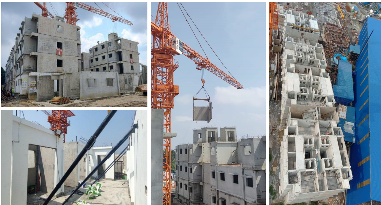
Fig.2: Erection of Precast Components
