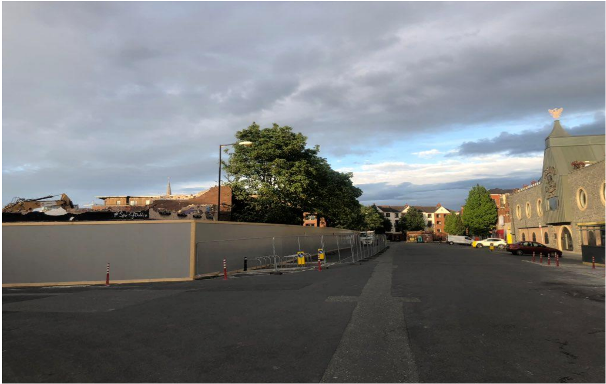
Fig 92: The beginnings of the demolition of Newmarket Square.
