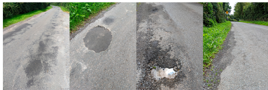
Figure 1. Photo images of several typical road surface defects were taken from the test road segment. From left to right, they show road surface distortion, patching, pothole, and rutting.
