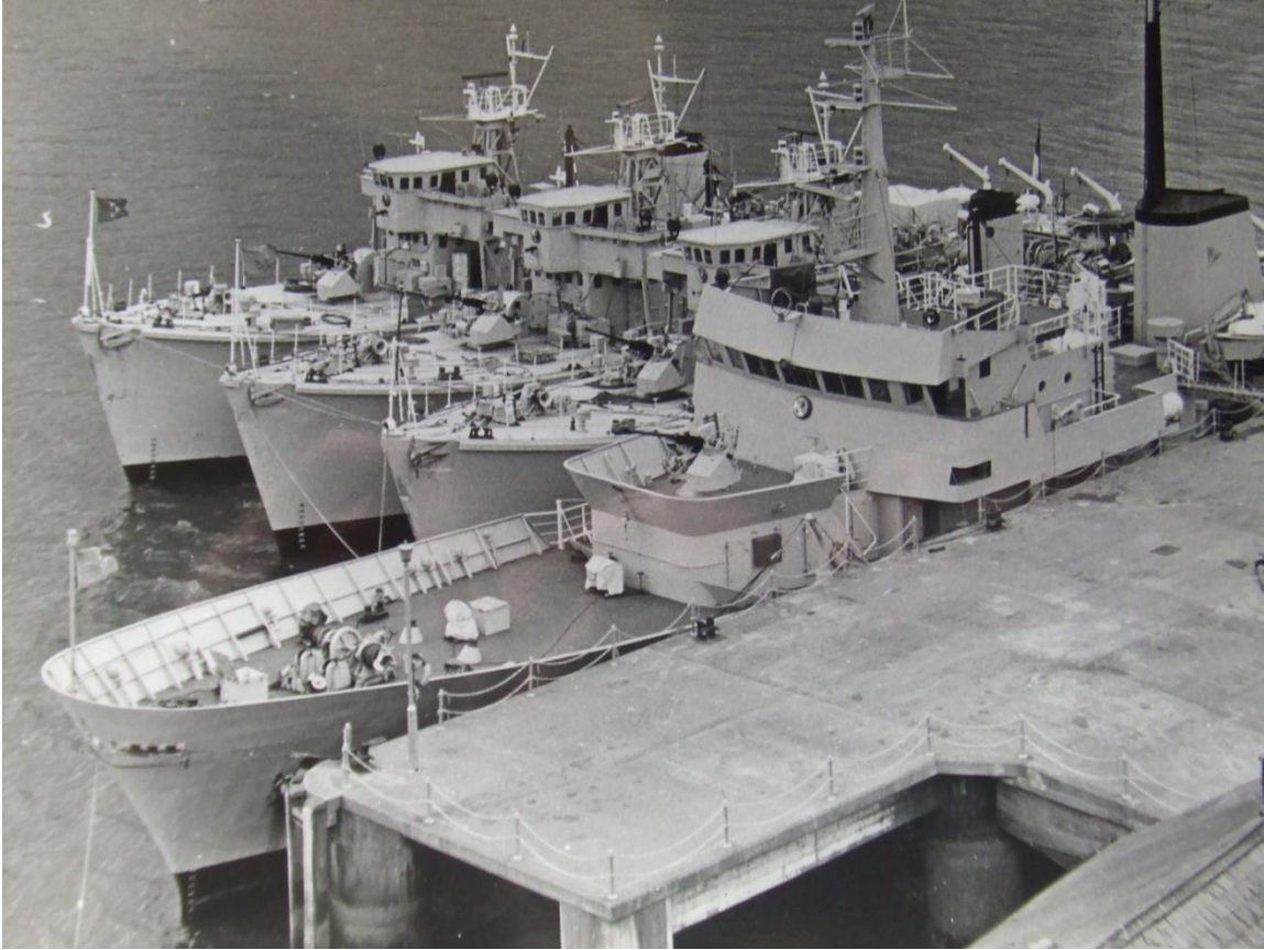
Fig 18: Coniston minesweepers alongside LE Emer .
