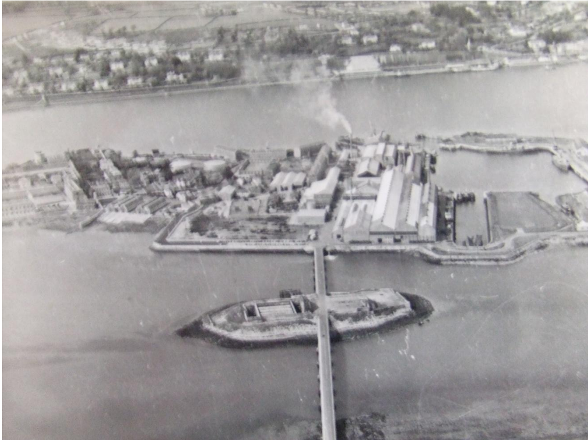
Fig 10: Aerial shot of Haulbowline.
