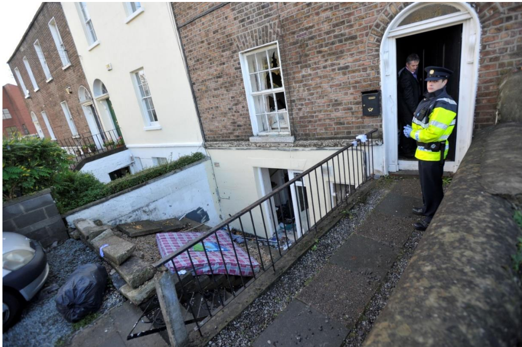
Figure 1. Entrance to Celia de Jesus's basement flat after the 2011 flood event.
