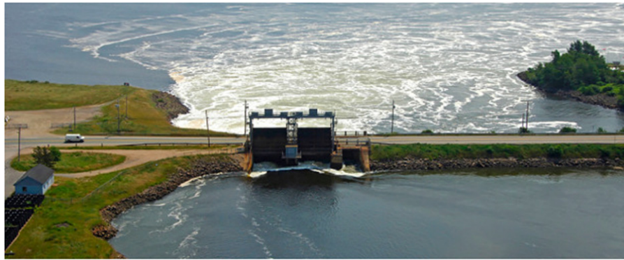
Fig. 4 The Annapolis tidal barrage, generating on the ebb tide. From (Khare et al. , 2018).
