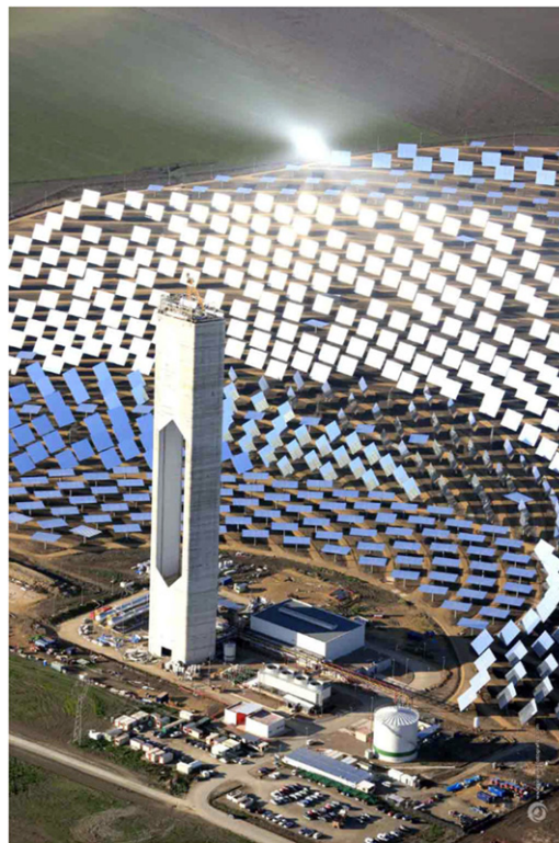
Fig. 13 20 MW thermodynamic solar plant near Seville ( Camacho and Berenguel, 2012 ).
