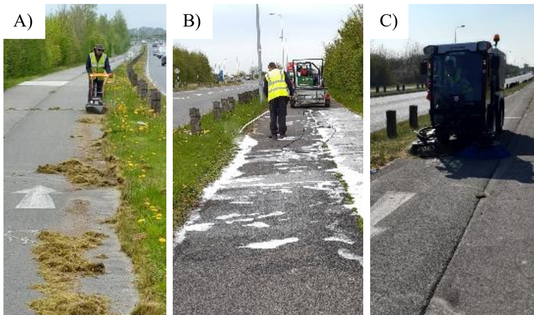
Plate 5-2 Mechanical and thermal experiments on the Millenium Link Road. The WeedHex machine (A), Hot Foam (B) and the Multihogg machine (C) treating the grass verge along the Millennium Link Road.
