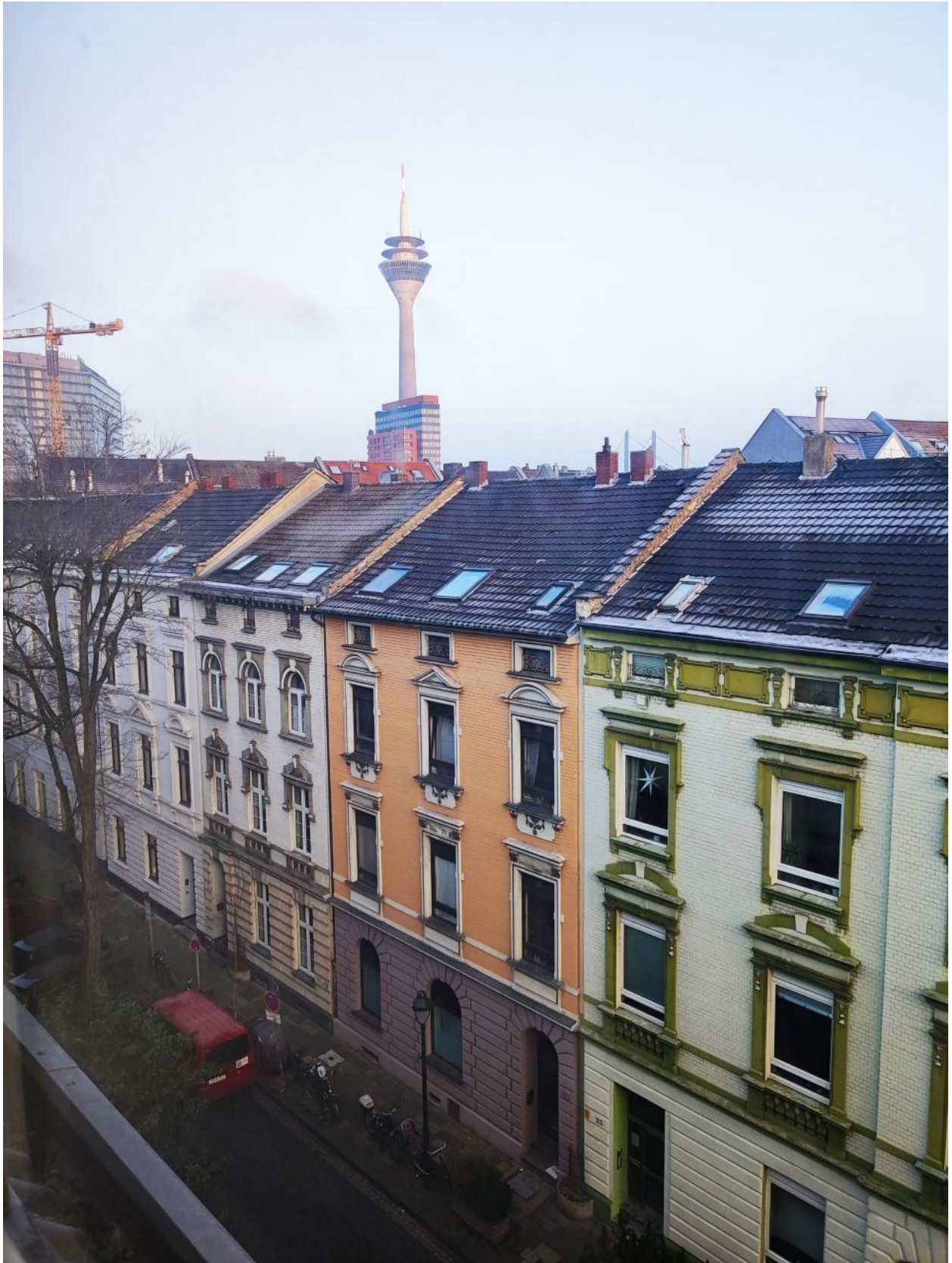
FIGURE 23 HOUSES IN A SIDESTREET IN DÜSSELDORF, GERMANY - DIFFERENT BUT HARMONIOUS AND ATTUNED. PHOTOGRAPH: ALAN XUEREB.
