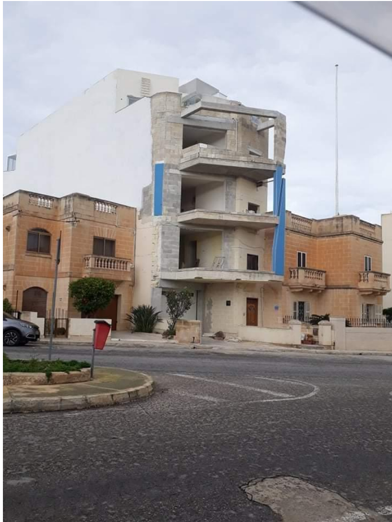
FIGURE 18 MOSTA, MALTA NEARNESS IS NOT SOLELY PHYSICAL IN HEIDEGGER'S VIEW BUT IT IS CONCEPTUAL, PHOTOGRAPH: ALAN XUEREB.
