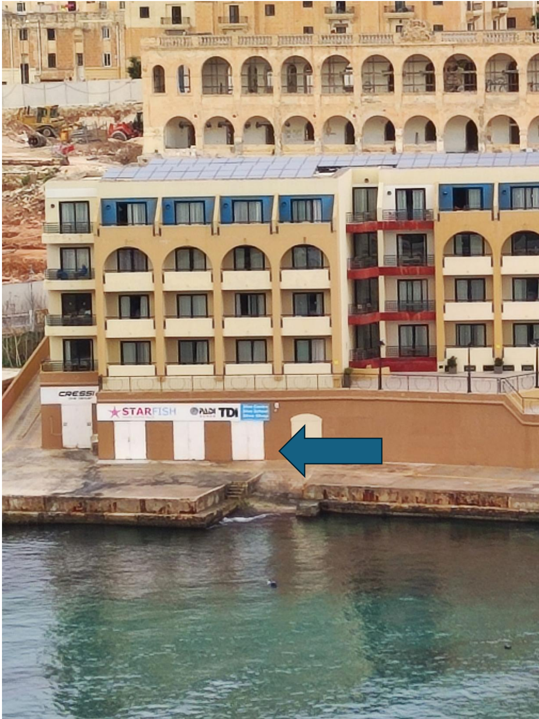
FIGURE 6 CORINTHIA MARINA HOTEL, ST JULIANS, MALTA RESPECTING THE OLDER ARCHITECTURE IN THE BACKGROUND WITH ONLY ONE ISSUE THE MARKETING OF COMPANIES STANDING OUT IN ORDER MAXIMISE THEIR EXPOSURE AND PROFITS. PHOTOGRAPH: ALAN XUEREB
