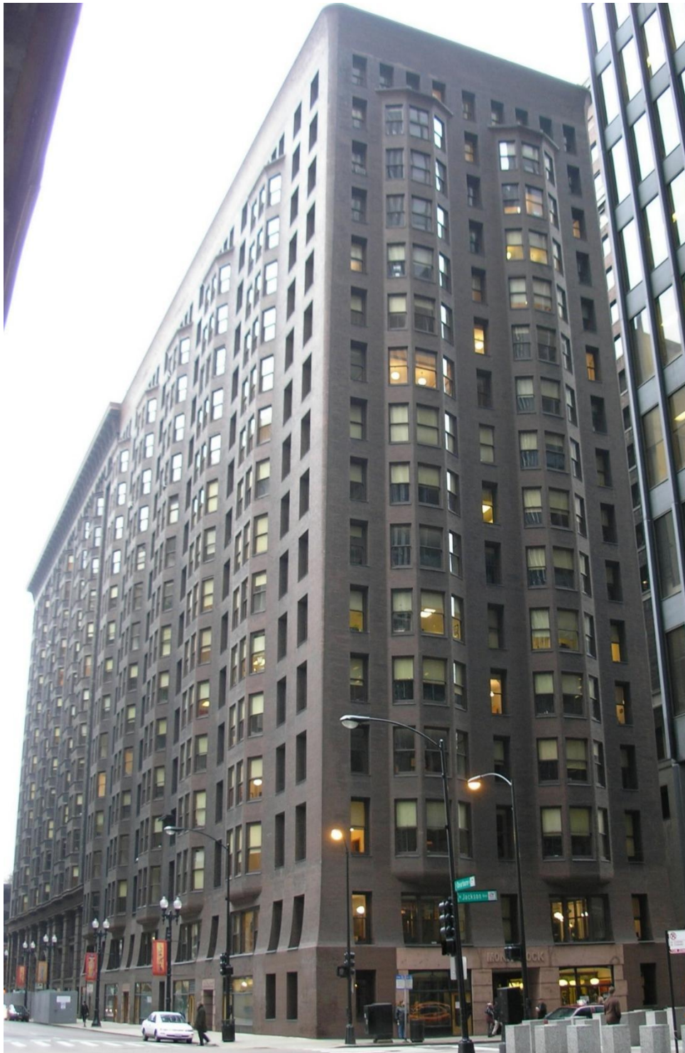
FIGURE 14 THE MONADNOCK BUILDING, 53 WEST JACKSON BOULEVARD, CHICAGO, ILLINOIS, SEEN FROM THE EAST SIDE OF JACKSON AND DEARBORN STREETS LOOKING SOUTH. PHOTOGRAPH: DAVID K. STAUB CREATIVE COMMONS ATTRIBUTION.
