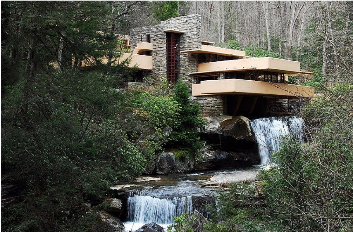
FIGURE 23 FALLINGWATER AT MILL RUN, PENNSYLVANIA, FRANK LLOYD WRIGHT. PHOTOGRAPH: LACHRIMAE72, WIKIMEDIA COMMONS
