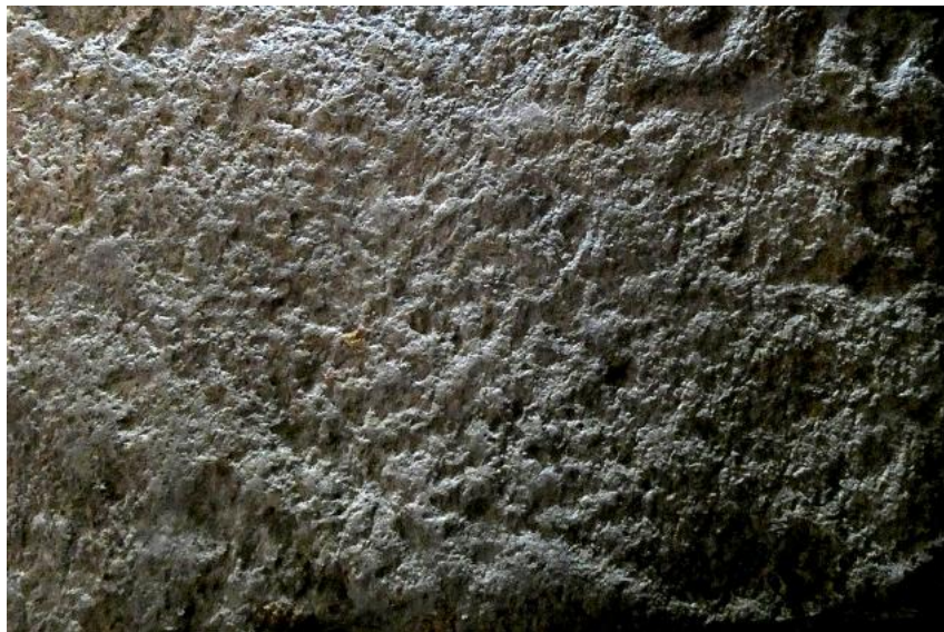
Fig. 16: BRN1, bush-hammered surface detail.
