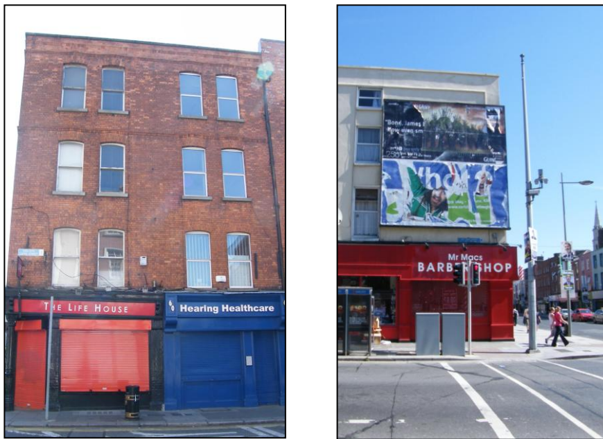
Figure 1.2 The current buildings that occupies the location of Thomas Sherrard’s residence/survey offices at 60 Capel Street (L) (1783-1800) and 1 Blessington Street (R) (1801-1828) (taken by F. O’Cionnaith, 2009).
