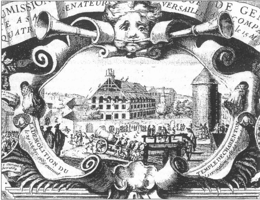
Figure 2: Demolition of Charenton Temple (BNF Estampes 72 C 52499 - by permission)
