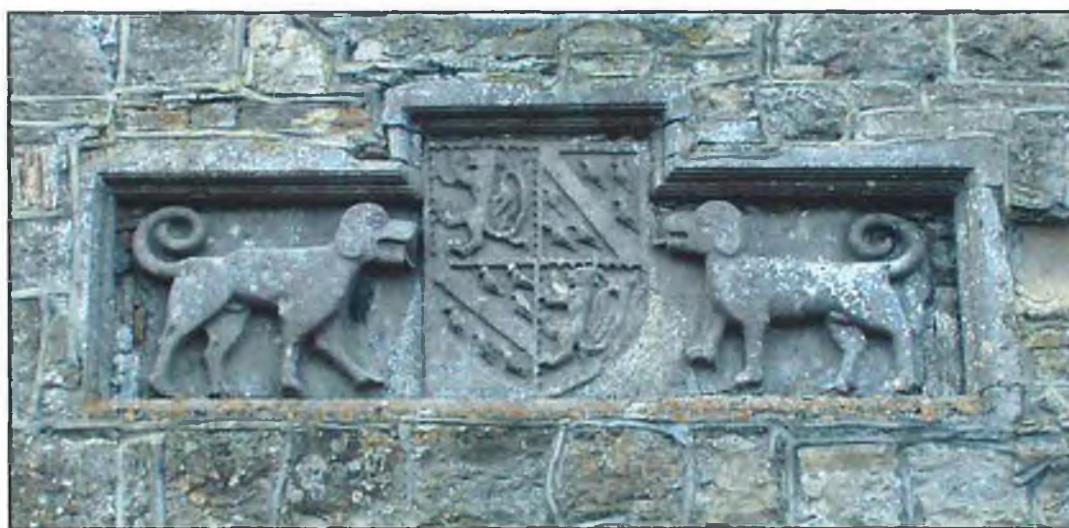
FIG. 9.2 Plaque on north wall at west end of Talbot’s Castle.
