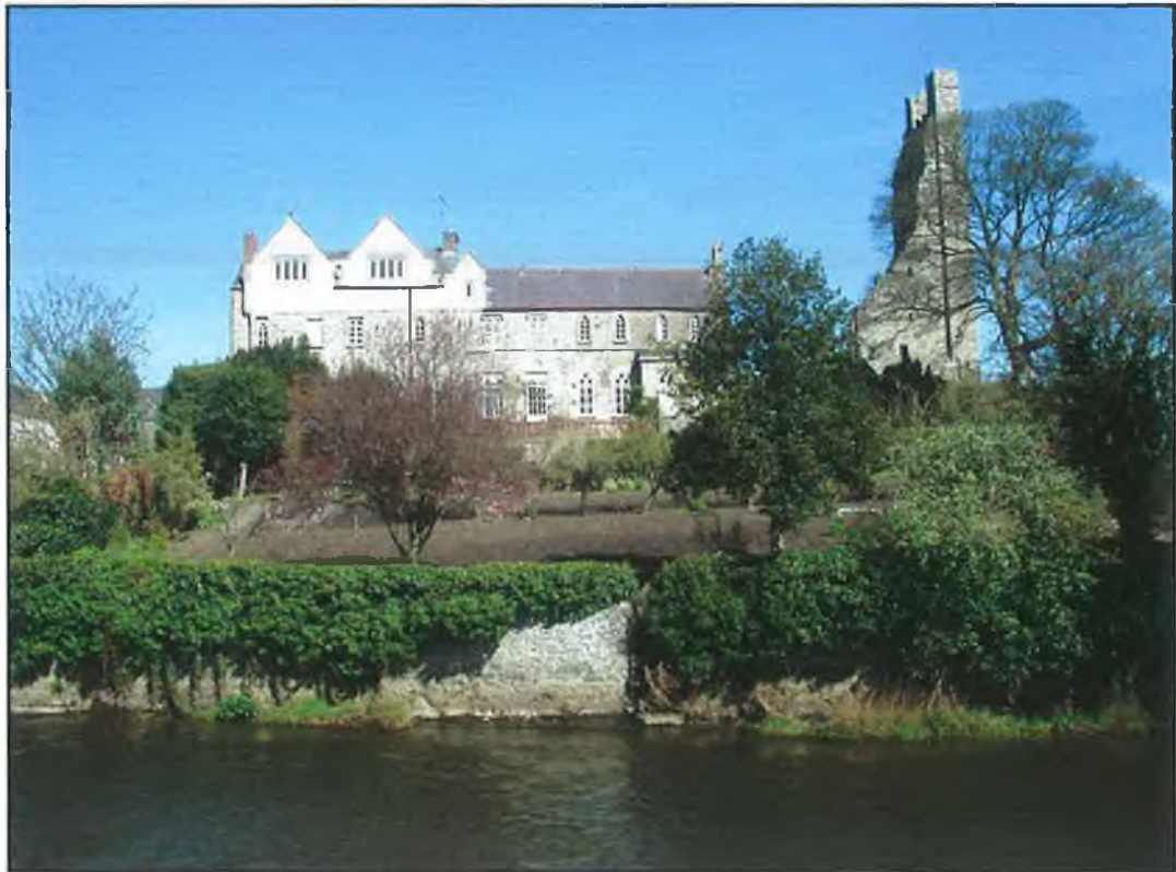
FIG. 9.1 Talbot's Castle. South façade, with Yellow Steeple to the east.
