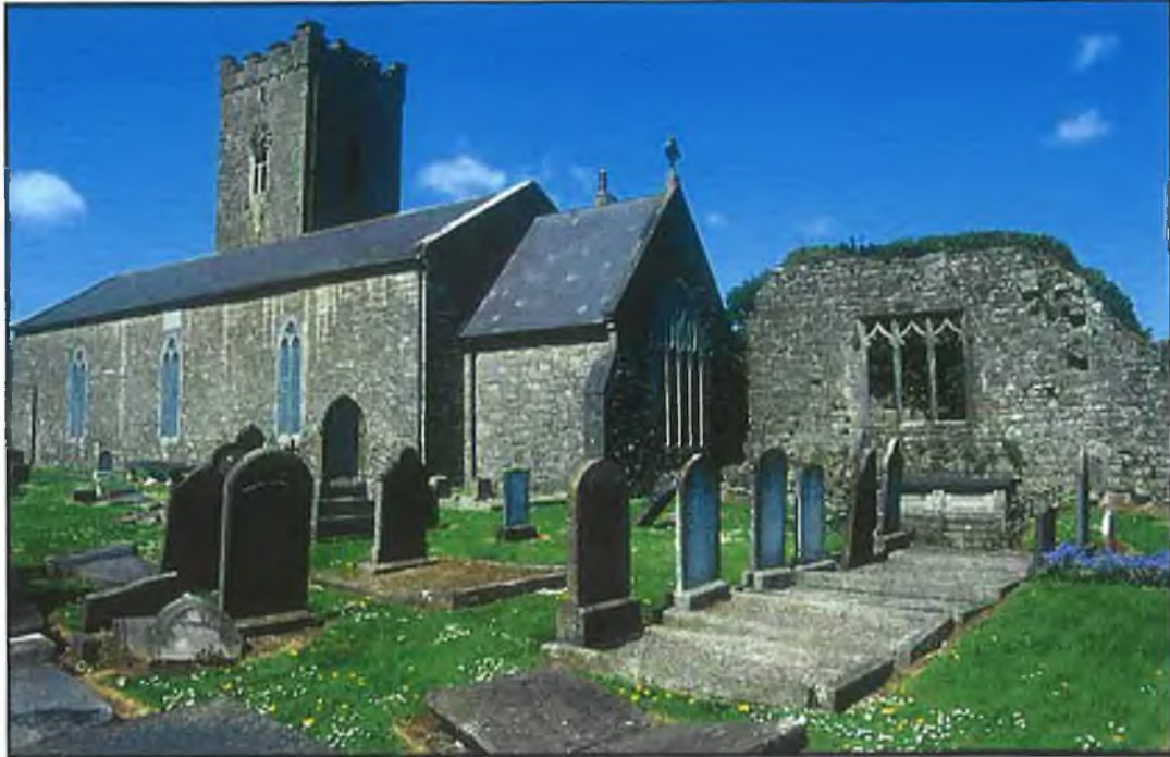
FIG. 7.1 General view of St Patrick's Church, Trim, from southeast.
