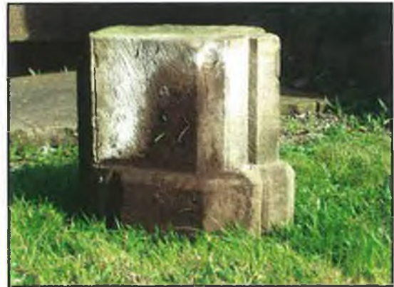
FIG. 7.28 Piece of door frame stored in chancel.
