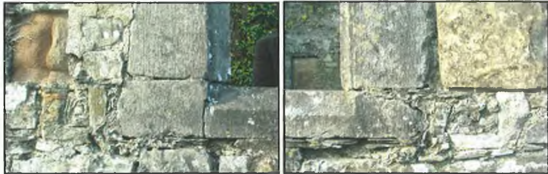
FIG. 7.7 The basal corner stones of the earlier window can be identified to the left and right of the present chancel window.
