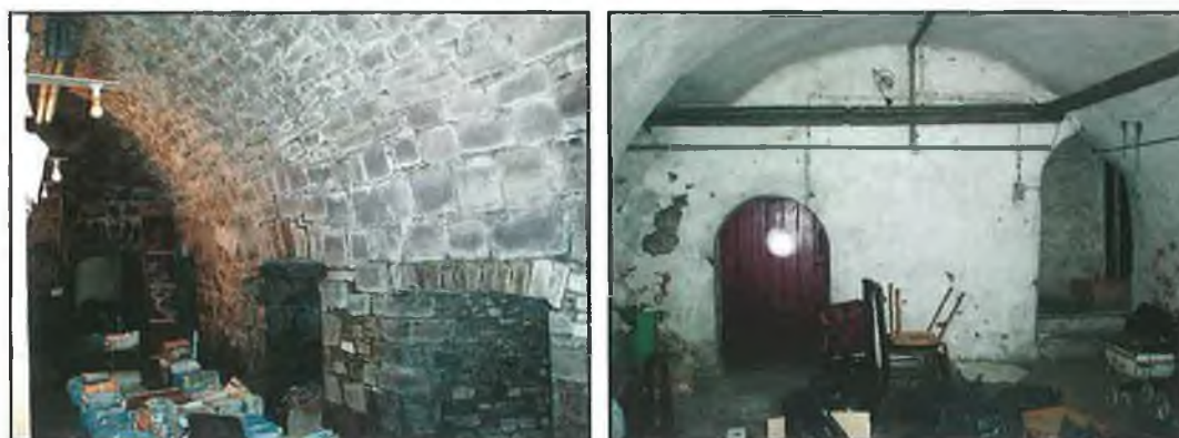
FIGS 8.10-11 The vaulted basement of Talbot's Castle.
