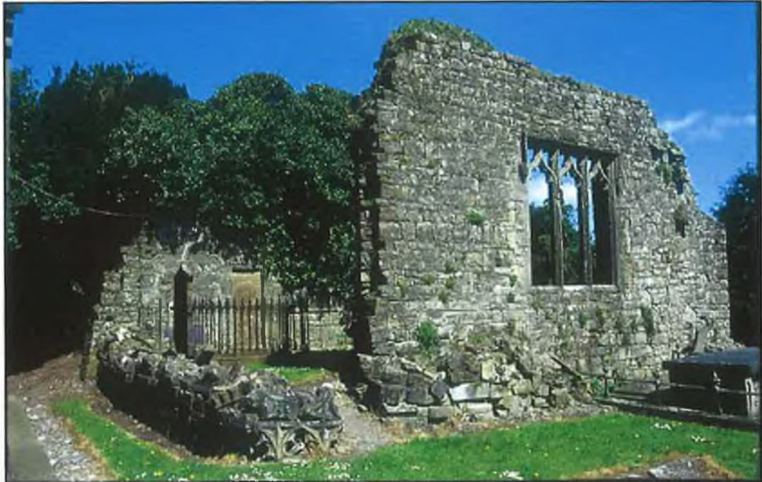
FIG. 7.5 Medieval chancel viewed from southwest.
