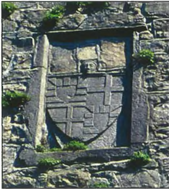
FIG. 7.4 Armorial shield in west wall of tower.
