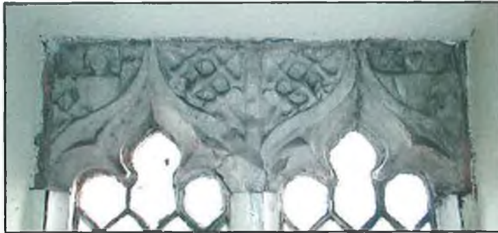
FIG. 9.9 Interior of cusped ogee heads on one of the second floor windows
