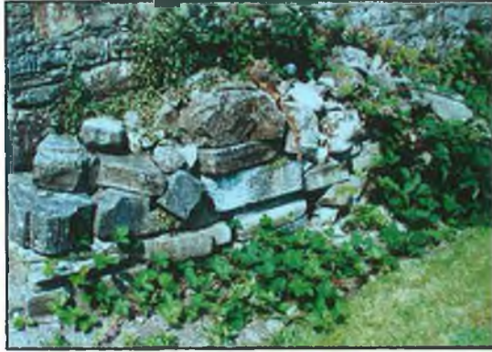
FIG. 7.22 Miscellaneous fragments of medieval masonry stacked beside chancel.
