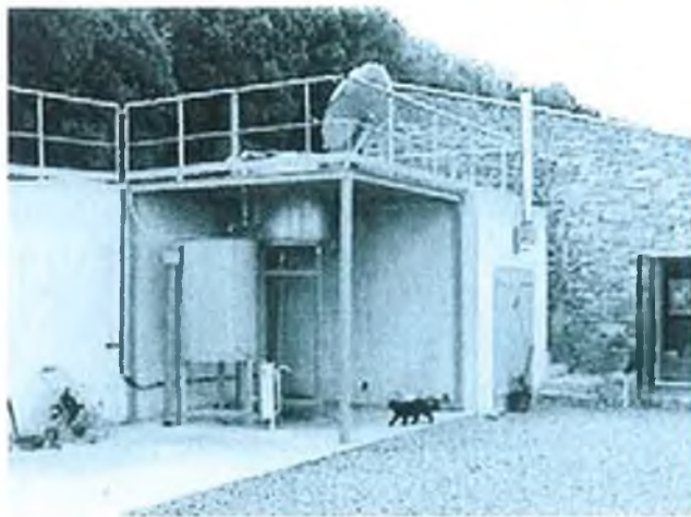
The tests are ok, the distillery is ready
