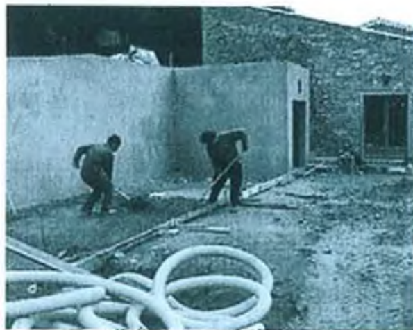
The construction of the buildi
