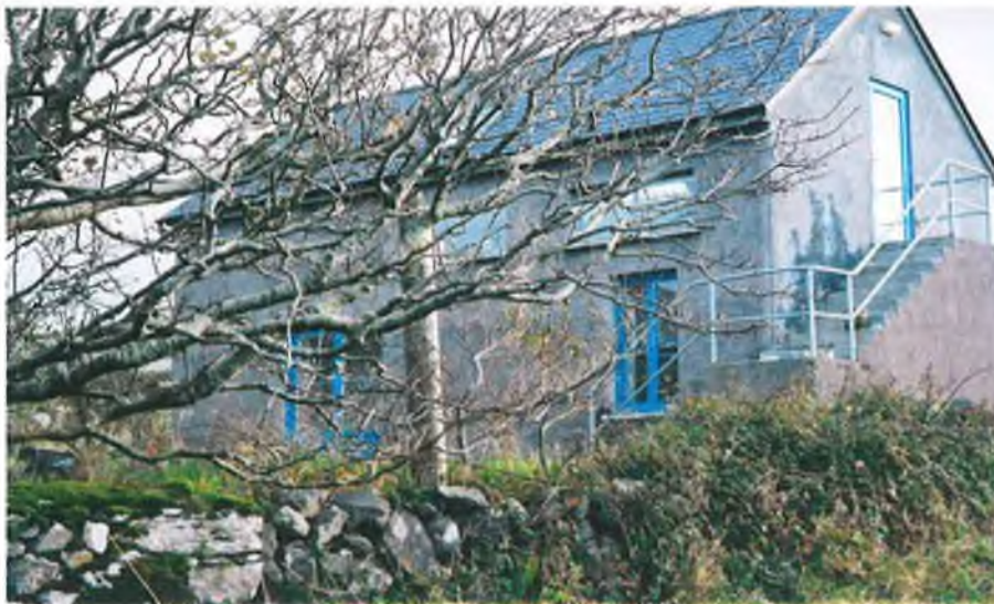
Fionuala's studio and bedroom. The concrete stairs lead to the studio, which features two velux's to the mountain side. Access to her bedroom on the ground floor, is gained through the double doors, featured to the left of the photograph.
