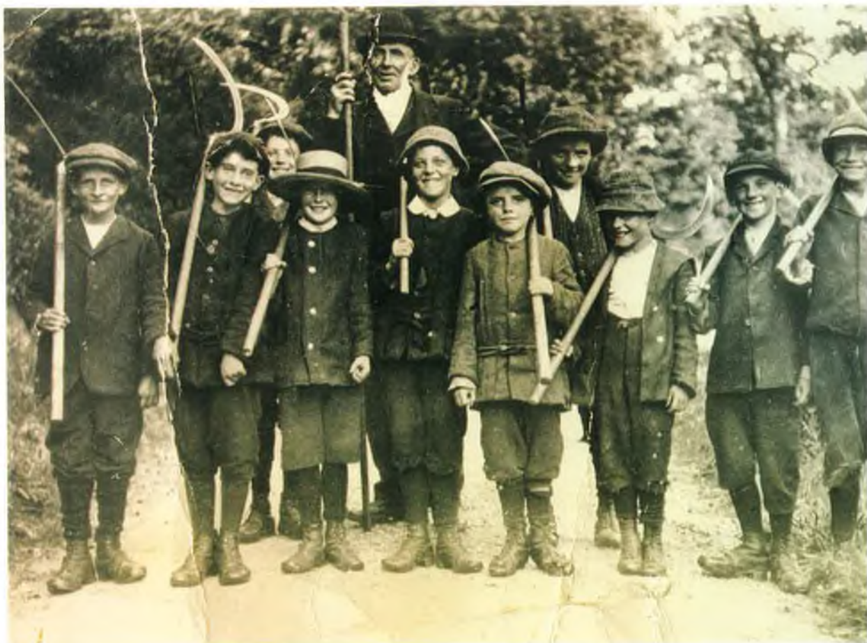
Plate 4. Young local workers preparing for thistle cutting at Carton estate, c.1910. Photograph courtesy of Bridie O'Brien
