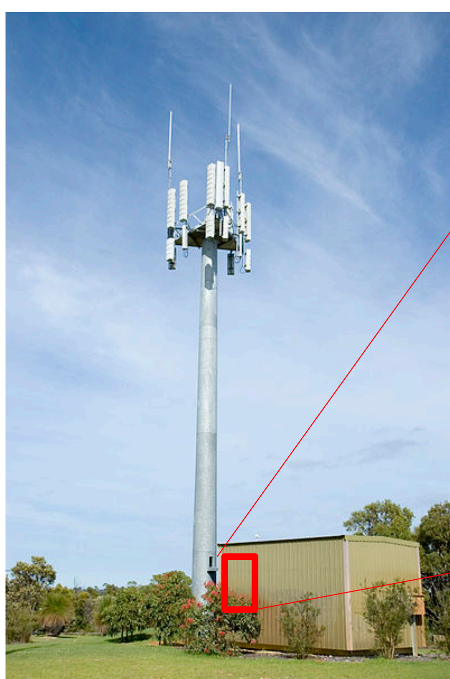
Fig 1. Location of a power amplifier in a base station
