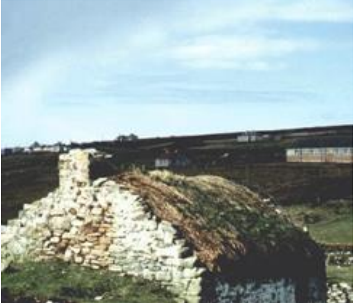
Plate 40: An Old Stone and Thatched House in Carrowteige Built Up Against an Earth Bank for Protection from Weather
