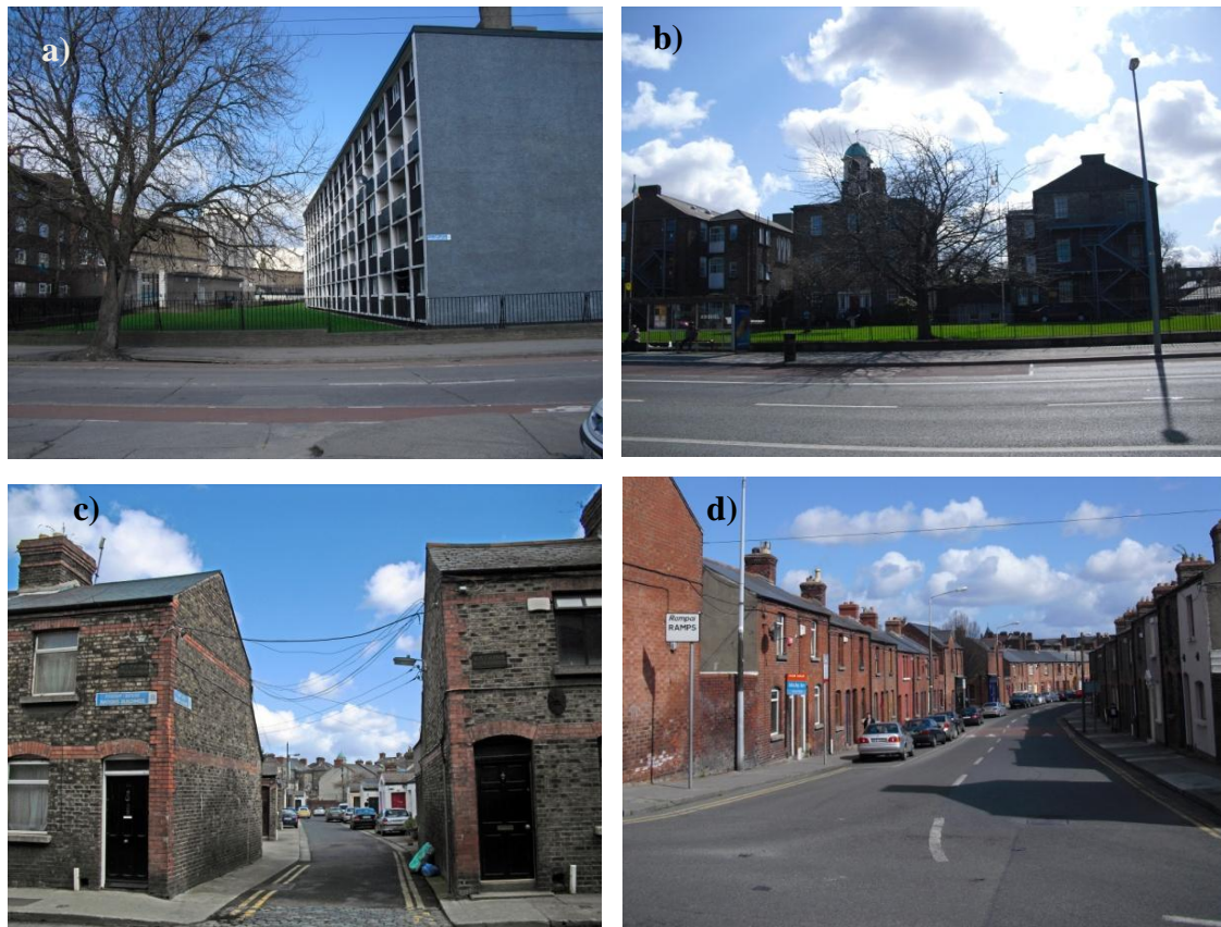
Figure 5.16 Land use in the surrounds of the EC site comprising of a) 4-5 storey apartment buildings, b) institutional buildings, and c) and d) 1 and 2 storey residential dwellings.
