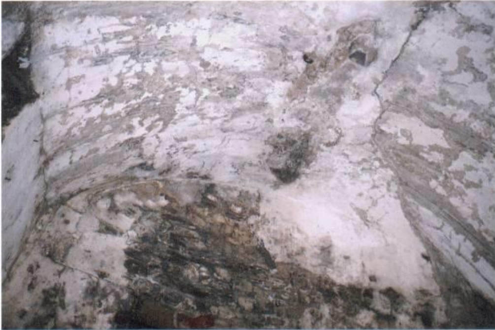
Plate 9 domed ceiling Plate 10 ground floor rooms
