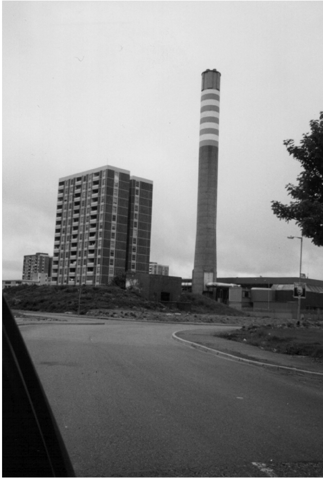
Fig. 2. Ballymun's tower blocks and the central power station. Heating on the old estate was turned on and off by the central power station: Residents could not even control the temperature of their own homes! Source: M. Boyle (May 2004).
