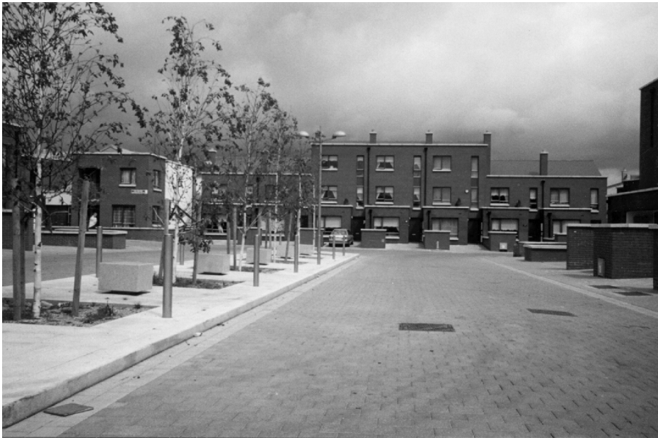
Fig. 4. Urban design and community building in Ballymun—new living quarters. Source: M. Boyle (May 2004).
