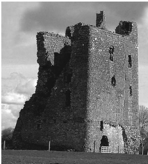
Figure 1. Rattin Castle Tower House, County Westmeath, Ireland.
