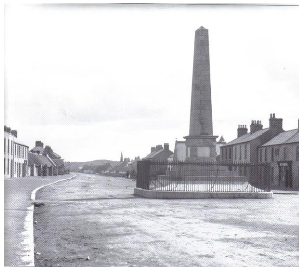
Plate 2, Holmpatrick Monument, Strand Street, Skerries (looking south). 2
