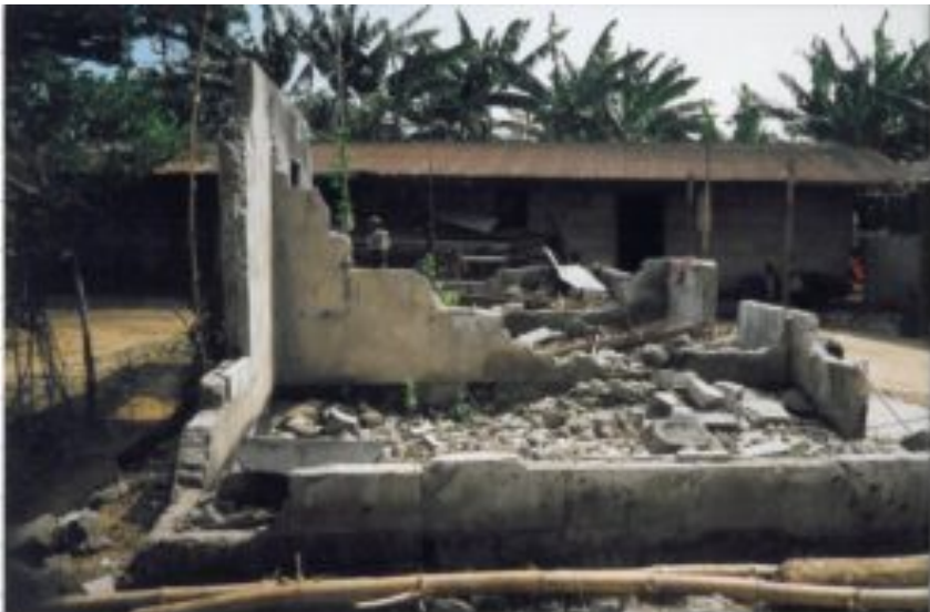
Destroyed buildings at Kaa Market in Ogoniland, 1994. Photograph by Mary Sweeney. Maynooth University Ken Saro-Wiwa Archive.
