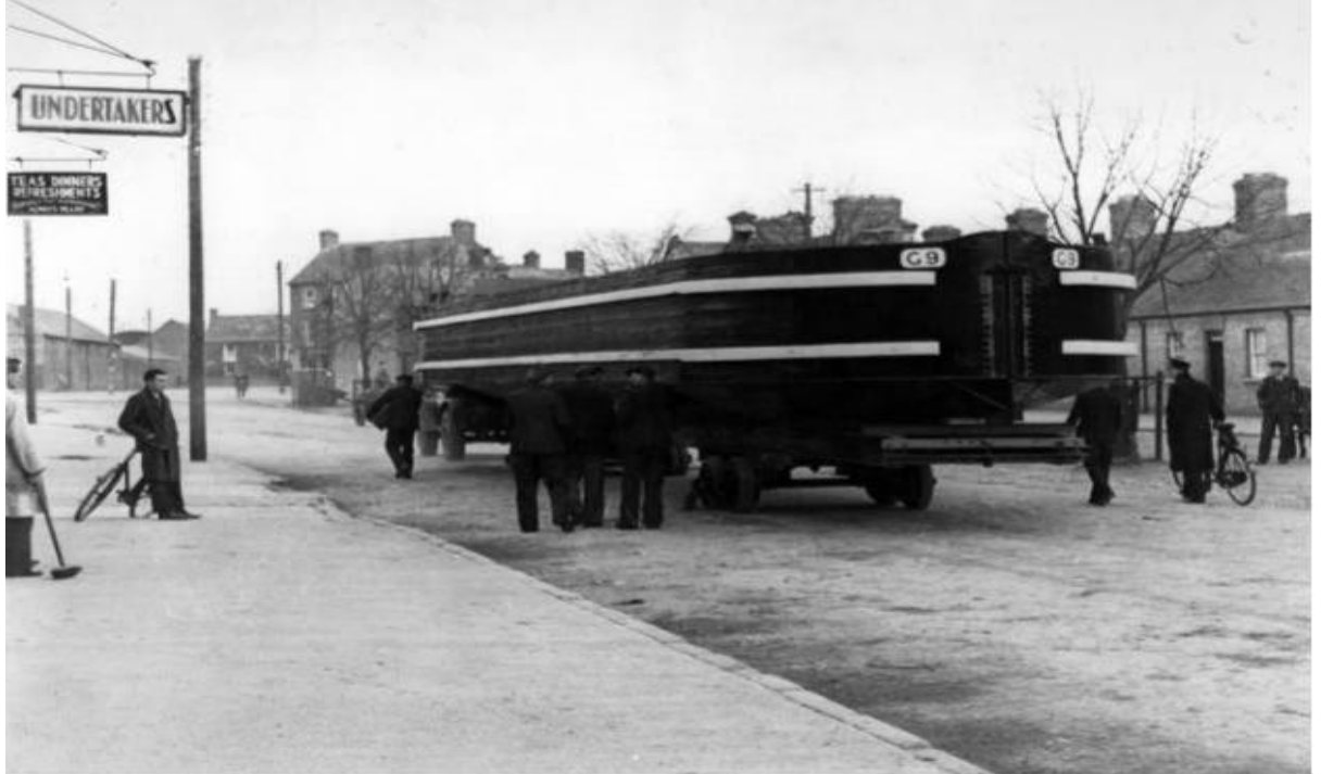
Figure 2.6 G-boat no. 9 being transported through Barrack Street, Carlow, 1941-45
