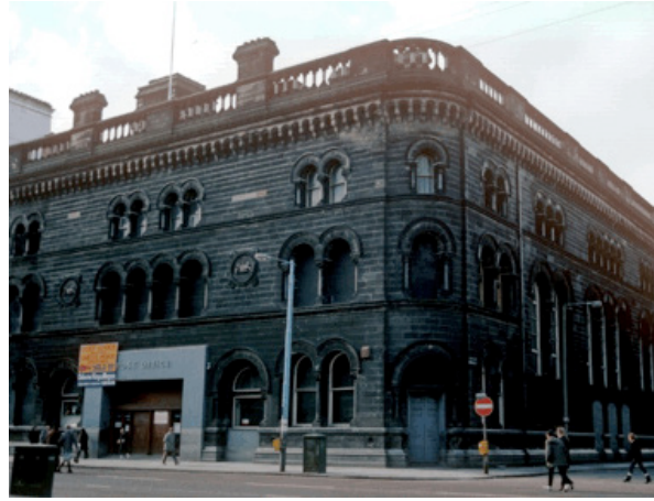
FIGURE 5 The Head Post Office in the mid-1980s prior to demolition.
