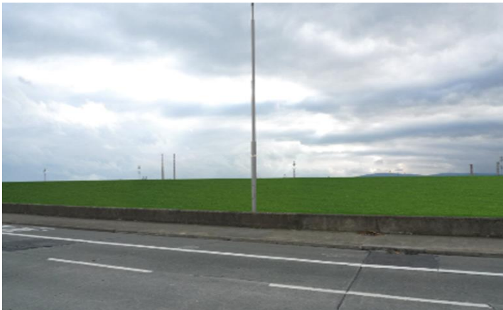
Figure 4.1: View of Clontarf promenade. Top - existing view. Bottom - virtual depiction of proposed flood defences along Clontarf promenade. Source: Dublin City Council (2011b)
